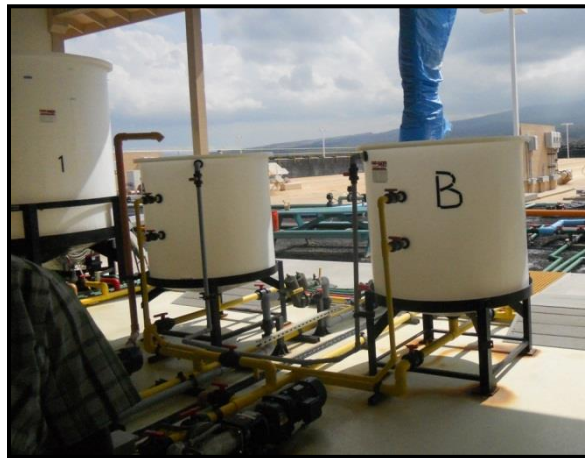
Figure 47. Photo of sedimentation tanks at Cellana facility taken by HNAABS team during fact finding trip to Hawaii.
