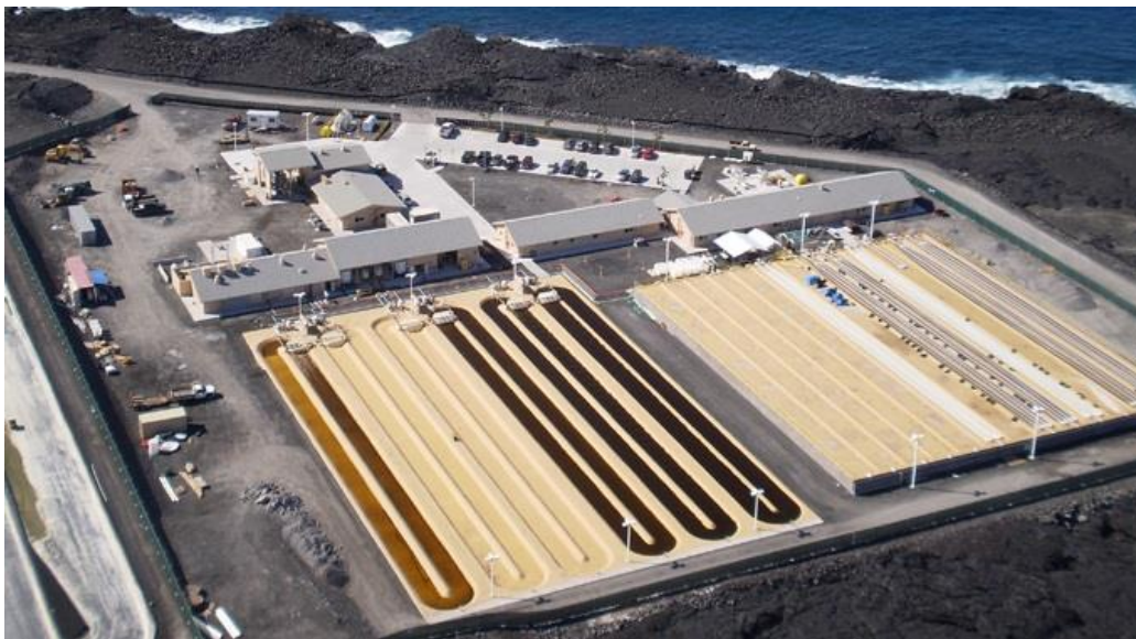
Figure 36. Algae farm demonstration facility in Kona, Hawaii utilizing hybrid growth method with photobioreactors (right) and open pond systems (left) (From Cellana 2013).
