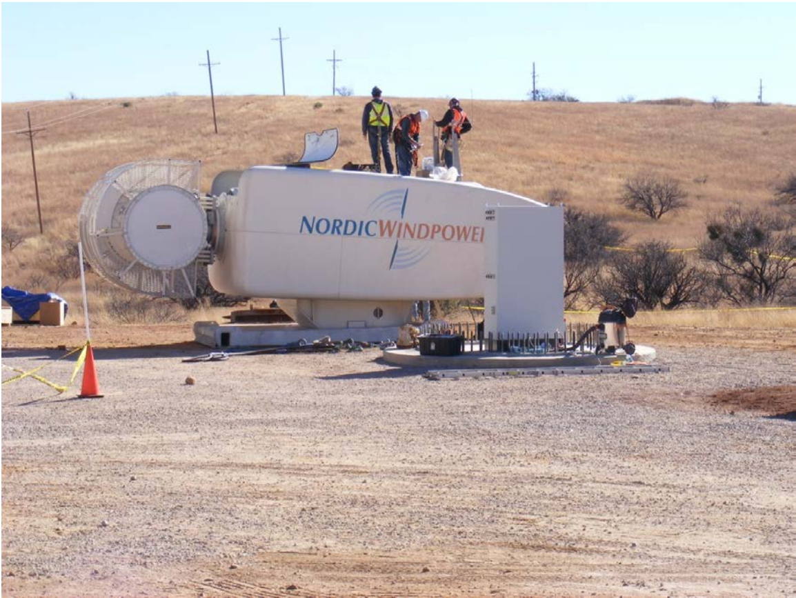
Figure 42. Nacelle on the Ground, Being Prepared for Mating of the Blades and Lifting
