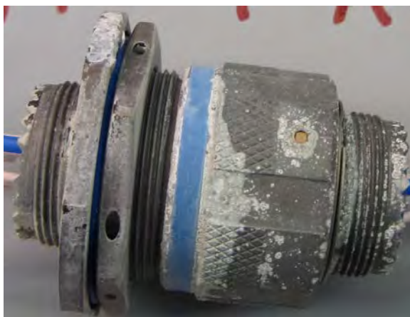
Higher Cad corrosion rate – discoloration on plug
