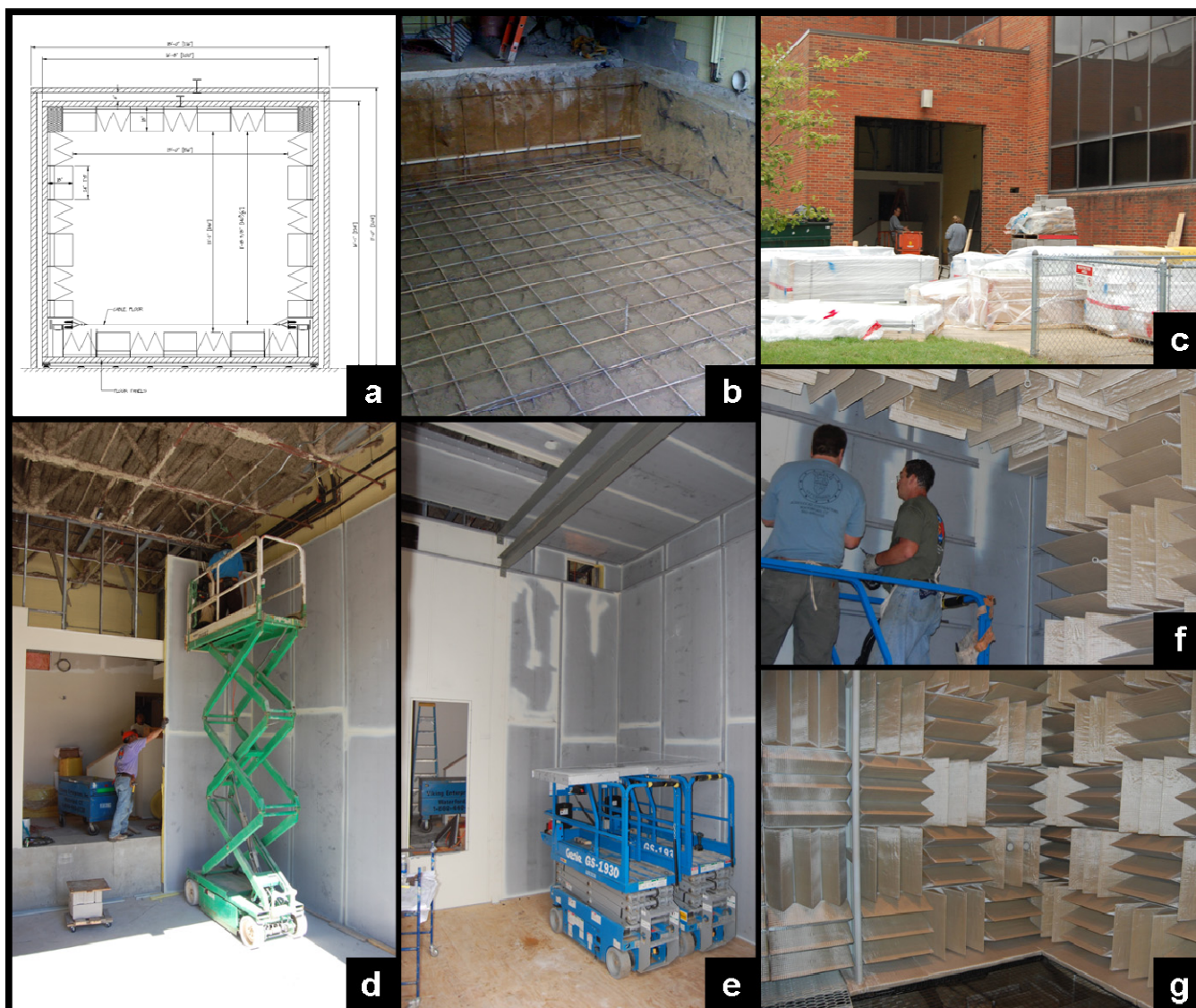
Figure 1. Anechoic chamber design and installation. a. Elevation drawing of anechoic chamber. b. Foundation preparation at Strickler Hall site on the University of Louisville Campus. c. Delivery of chamber materials. d. Installation of outer chamber walls. e. Installation of inner chamber walls. f. Installation of sound absorbing wedges (18-inch depth). Chamber installation was performed by Viking Enterprises, Inc (Waterford, CT). g. Completed chamber viewed from inside. Entrance door is visible on the left.
