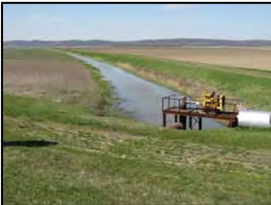
Figure 10.27.2 – L-488 site. Landside of levee inlet headwall and pump (top left). Riverside outlet with screw gates (top right). Top of levee looking landward (bottom left). Top of levee looking riverward (bottom right).
