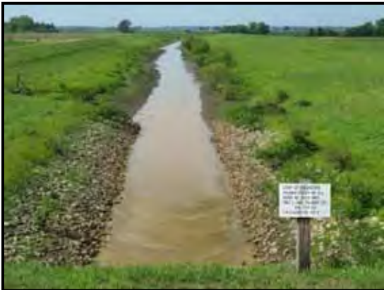
Figure 10.39.2 – L-246 Palmer Creek drainage through main levee. Inlet of box culvert (top left). Outlet of box culvert with flap gates and data logger on left structure wing (top right). Top of levee looking landward at inlet ditch; side ditch culvert on left side; tieback berms on either side of inlet ditch (bottom left). Top of levee looking riverward (bottom right).
