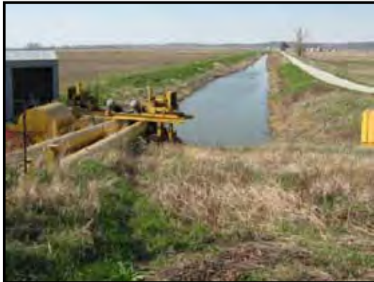
Figure 10.26.2 – L-497 Main Outfall site. Culvert inlet with three 60-in. CMPs, pump station, and landside data logger (top left). Concrete outlet gate structure with screw gates (top right). Top of levee looking landward (bottom left). Top of levee looking riverward (bottom right).
