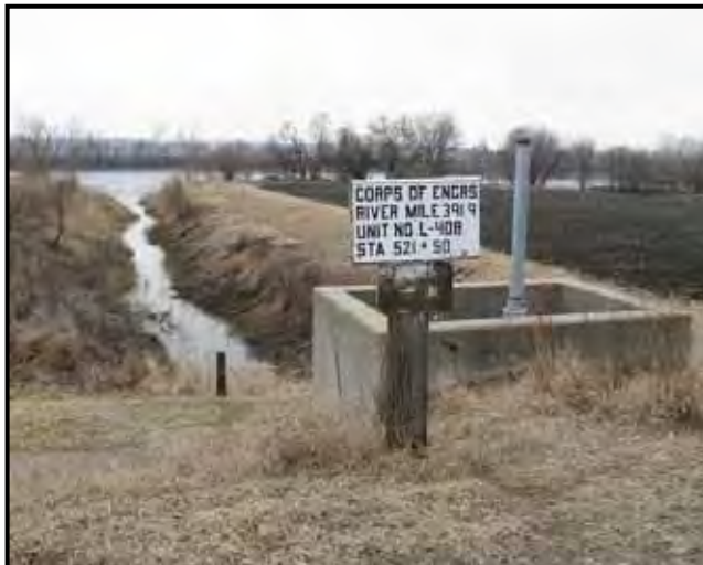
Figure 10.30.2 – L-408 site. Sensor pipe on 6-ft x 5-ft RCB culvert inlet headwall (top left). Outlet drainage ditch looking toward levee before DCP installation (top right). Top of levee looking landward (bottom left). Top of levee looking riverward before DCP installation (bottom right).
