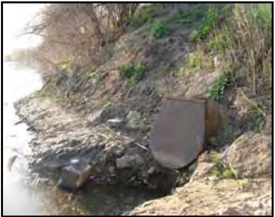
Figure 10.24.2 – Holt County LD No. 9 site and gages. Upstream culvert gage at inlet of 36-in. CMP (upper left). River gage (upper right). Flap-gated outlet on river (lower left). Inlet ditch and interior fields (lower right).
