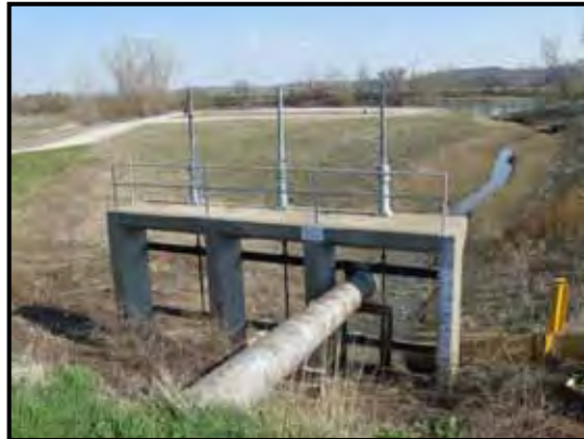
Figure 10.26.2 – L-497 Main Outfall site. Culvert inlet with three 60-in. CMPs, pump station, and landside data logger (top left). Concrete outlet gate structure with screw gates (top right). Top of levee looking landward (bottom left). Top of levee looking riverward (bottom right).
