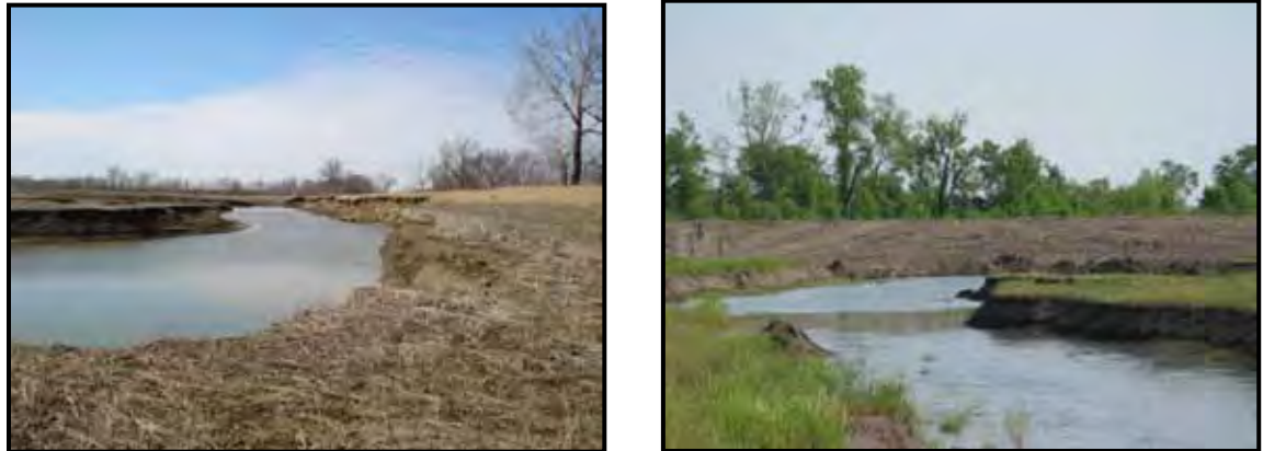
Figure 10.44.2 – Tebbets East LD site. 2008 levee blowout from back channel of Missouri River before repairs (left). Repaired levee blowout but interior washout still present in August 2009 (right).
