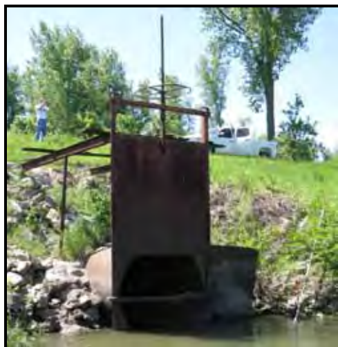
Figure 10.33.3 – MO Valley DLD gages. Landside data logger by slide gate inlet (left). River DCP located in Corps of Missouri River Area Office at Napoleon (left).
