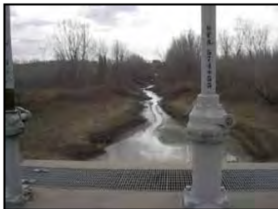
Figure 10.39.2 – L-246 Palmer Creek drainage through main levee. Inlet of box culvert (top left). Outlet of box culvert with flap gates and data logger on left structure wing (top right). Top of levee looking landward at inlet ditch; side ditch culvert on left side; tieback berms on either side of inlet ditch (bottom left). Top of levee looking riverward (bottom right).
