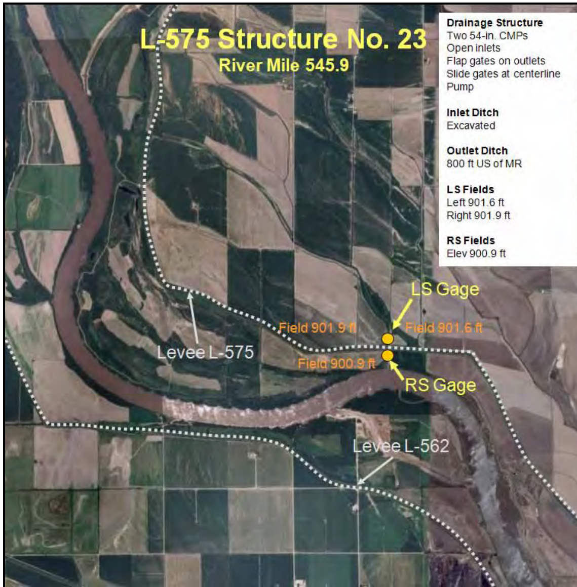
Figure 10.20.1 – L-575 Structure No. 23 location
