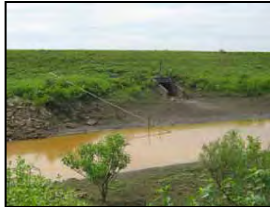
Figure 10.39.4 – L-246 Palmer Creek side ditch through tieback berm. Inlet for 36-in. culvert through tieback berm with datalogger (top left). Outlet for 36-in. culvert through tieback berm (top right). Stoplog structure at centerline of tieback berm (bottom left). Outlet of tieback levee draining to Palmer Creek with landside datalogger shown (bottom right).
