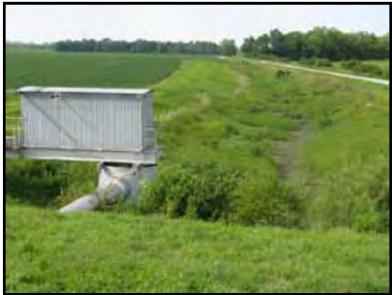
Figure 10.40.3 – Side ditch culvert through L-246 Dalton Ditch berm. Inlet of 48-in. culvert through right bank side berm with data logger (top left). Outlet of 48-in. culvert with flap gate (top right). Side ditch with pump station looking landward (bottom left). Dalton boat ramp looking downstream (bottom right).
