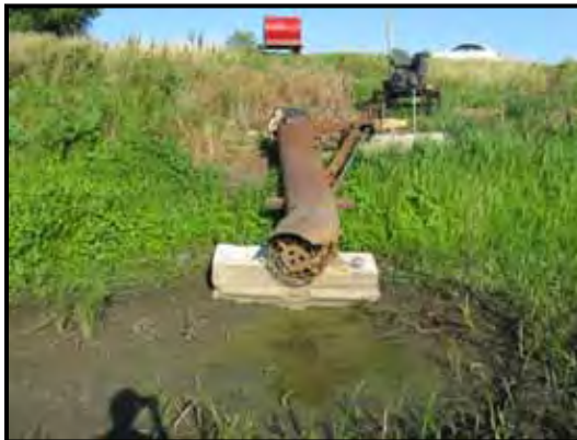
Figure 10.38.2 – Brunswick LD site. Landside 60-in. culvert inlet through main levee (top left). Riverside flap-gated outlet with pump station outlet pipe to left; flap gage controlled by pulley (top right). Top of levee looking landward at inlet ditch and pump station with engine (center left). Outlet ditch to mouth of Grand River (center right). Pump station with 24-in. inlet pipe (bottom left). Pump station outlet encased in section of scrap 60-in. CMP (bottom right).
