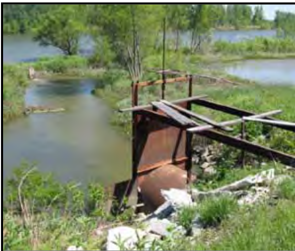
Figure 10.33.2 – MO Valley DLD site. Inlet slide gate and landside gage (top left). Outlet with flap gate and weight (top right). Top of levee looking landward at interior ponds and fields beyond (bottom left). Outlet drainage ditch (bottom right).
