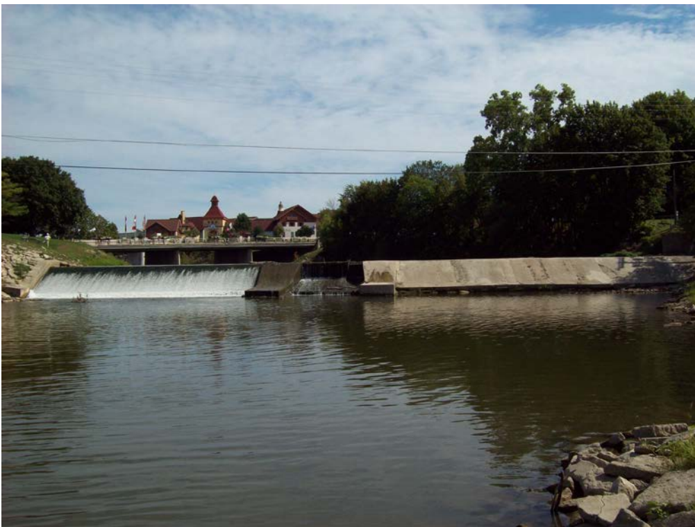
Figure 5: Overview looking upstream (southeast) at the Frankenmuth Dam (Fall 2008).
