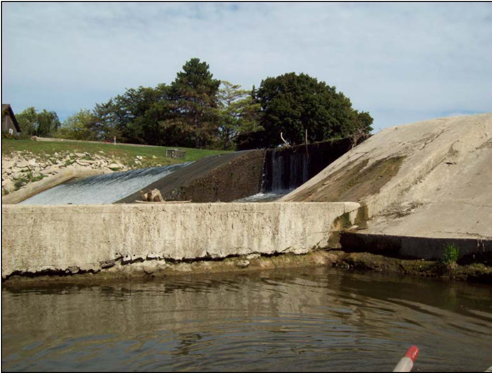
Figure 6: Looking northeast at the downstream face of the Frankenmuth Dam (Fall 2008).
