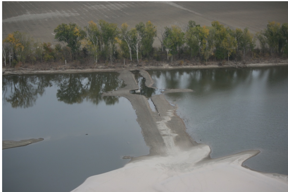
Cross levee between the upper and lower management areas blowout. Photo taken October 24, 2011
