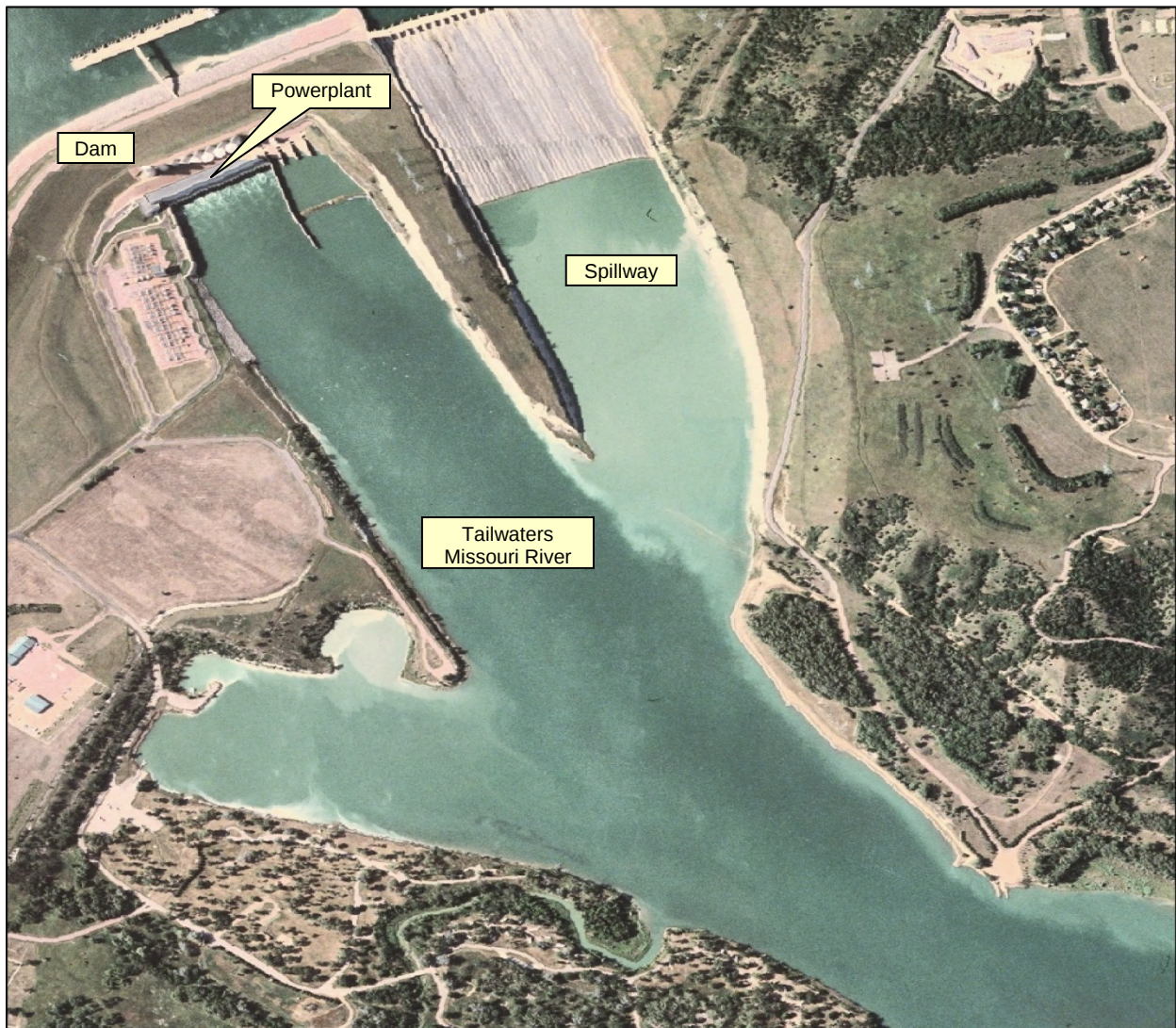
Aerial Photo of Fort Randall Dam Tailwaters
