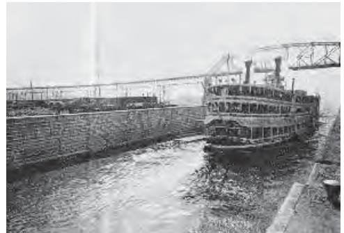
First vessel through L&D 26
