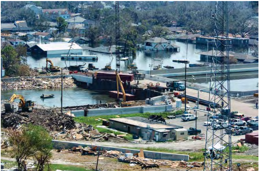
Construction of sheet piling on 17th Street
