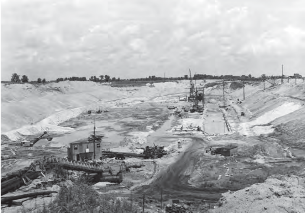
Chain of Rocks project cofferdam construction, 1947
