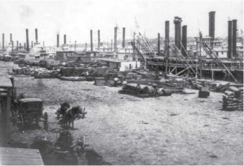
Levee, St. Louis, Missouri (LOC)
