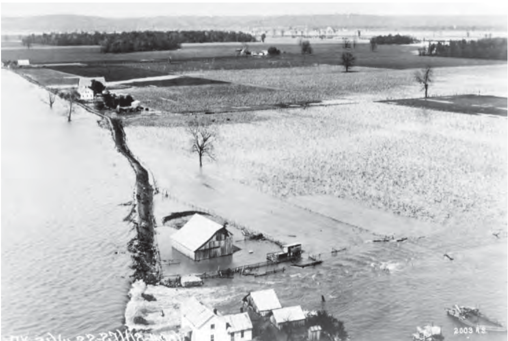
Grand Tower, Illinois, after levee break during 1927 flood
