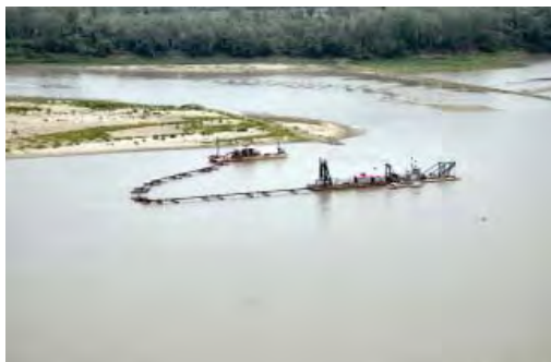
Construction of chevron dike
