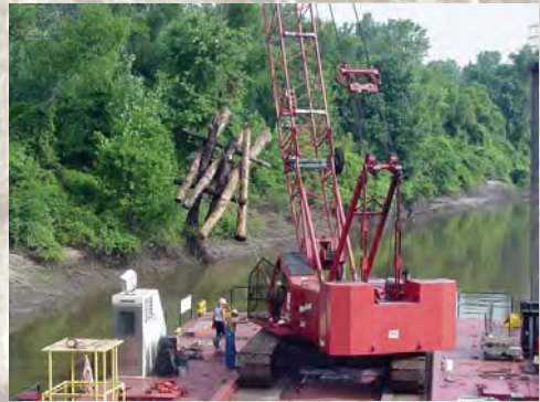
Woody structure being lowered into river
