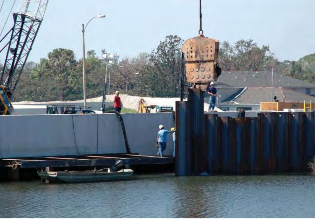
Sheet piling construction at canal in New Orleans after Hurricane Katrina
