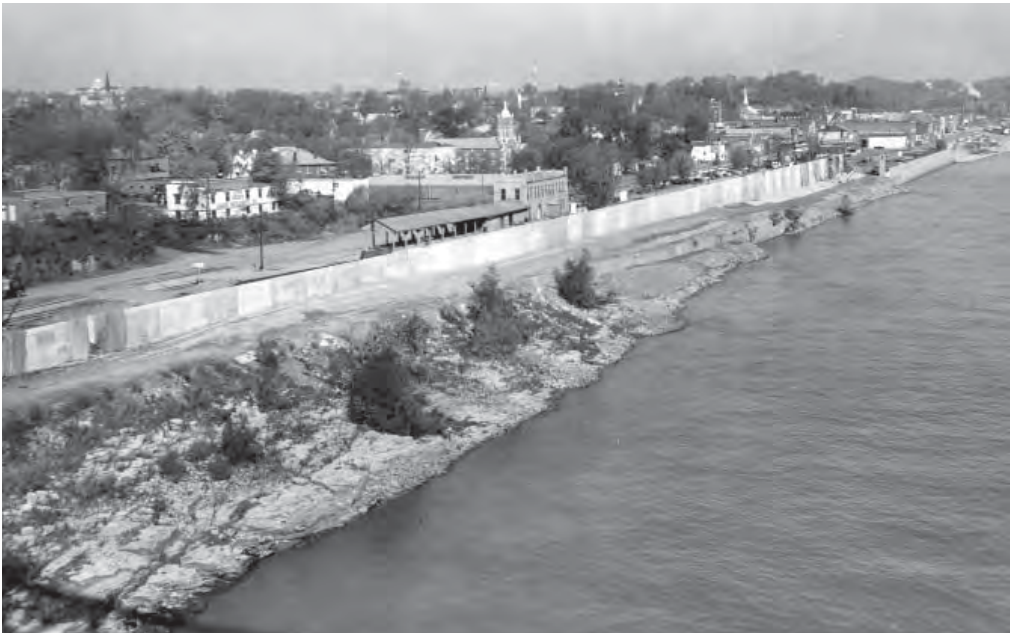
Cape Girardeau floodwall
