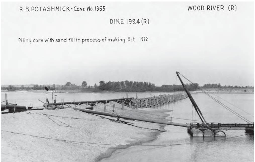
Early river training structure
