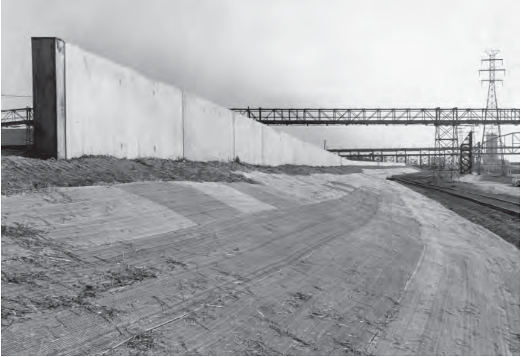
East St. Louis floodwall, 1951
