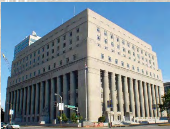
Federal Building at 12 Street (now Tucker Blvd.) and Market
