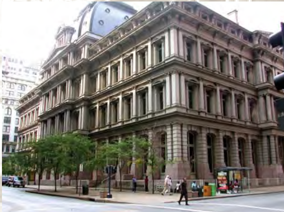
Old Post Office Building
