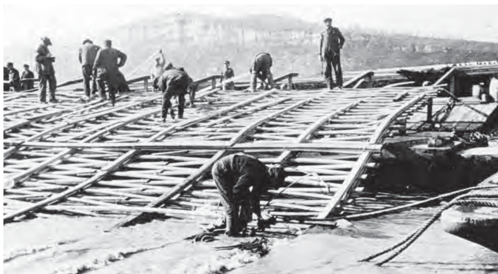
Construction of early mattress revetment
