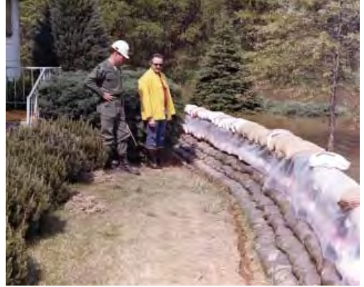
Sandbagging at Arnold, Mo. during 1973 flood
