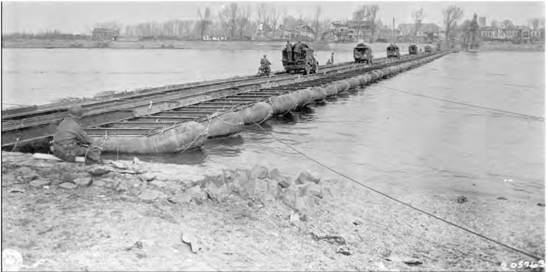
Engineers employing a pneumatic bridge in Europe during World War II. U.S. Army Engineer School.
