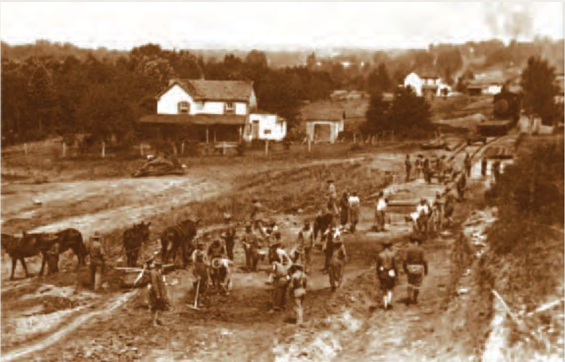
Engineers constructing a corduroy road as part of a training exercise at Camp Humphreys, Va., 1918. U.S. Army Engineer School.
