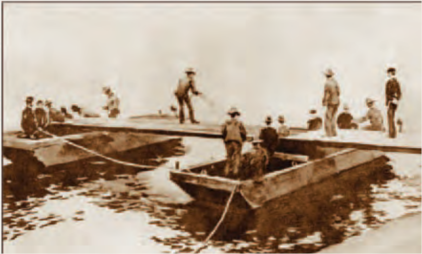
Students at Willets Point building a pontoon bridge, 1899. U.S. Army Engineer School.
