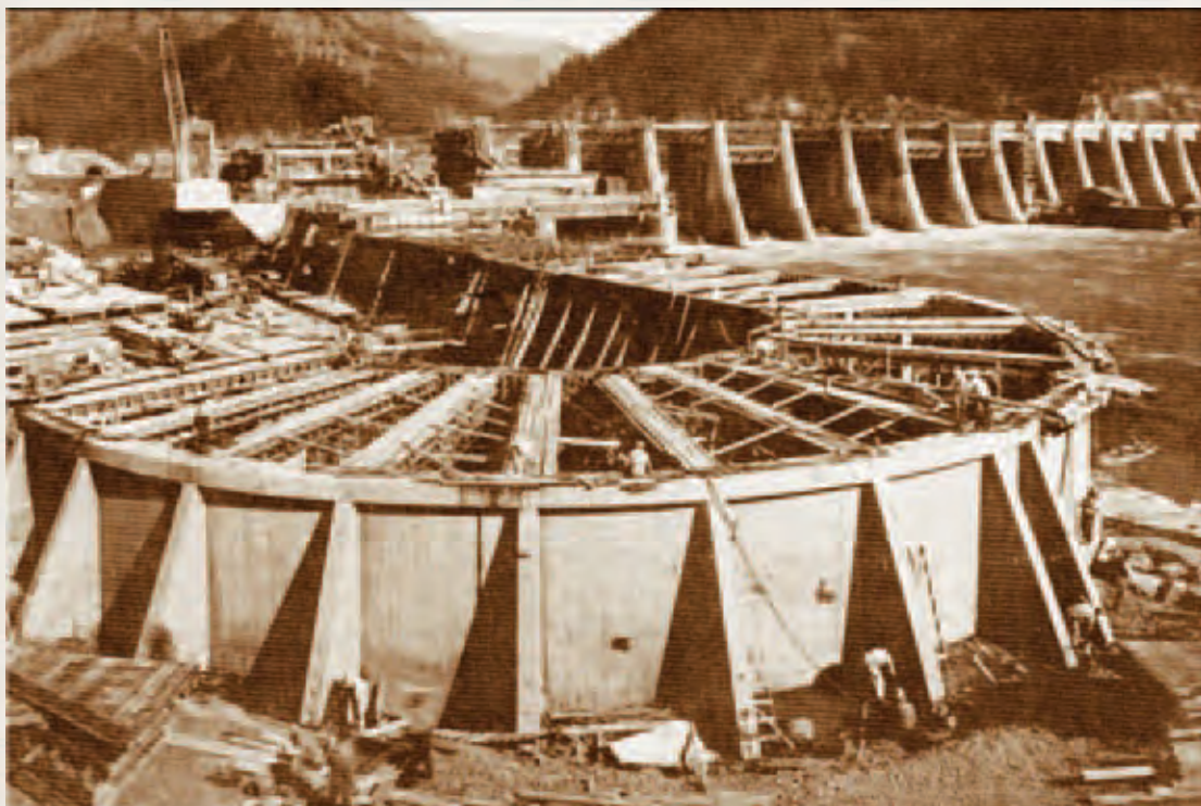
Bonneville Dam fish ladder under construction, 1937.
