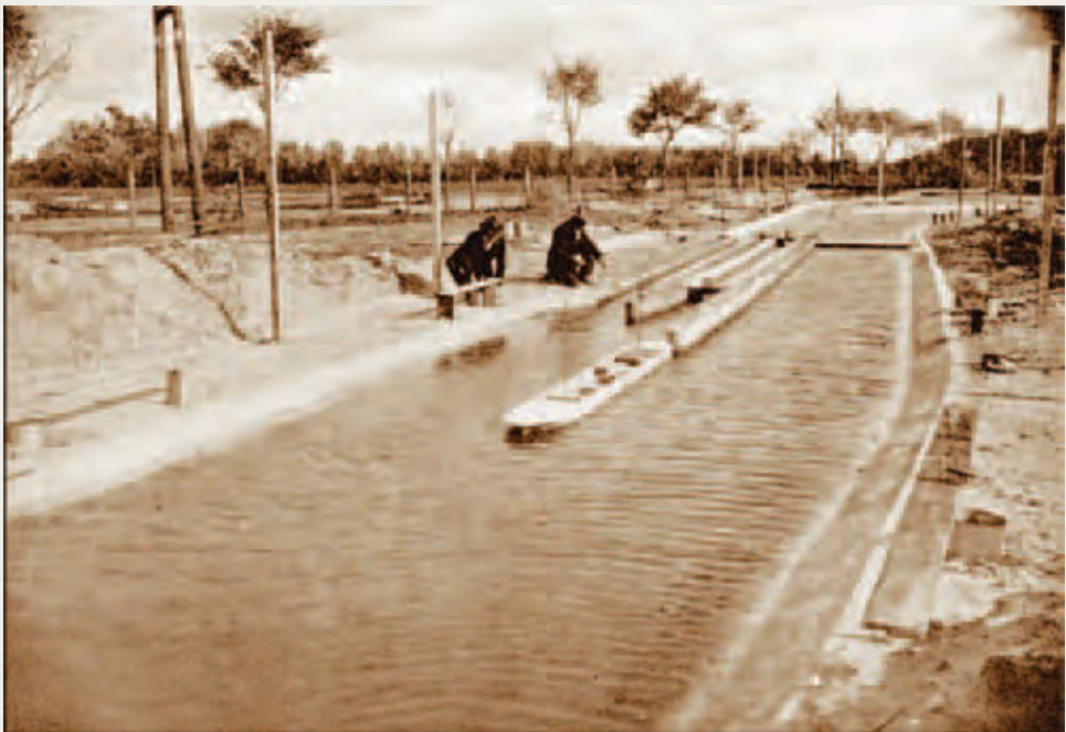
Outdoor hydraulic river model in Dresden, Germany.
