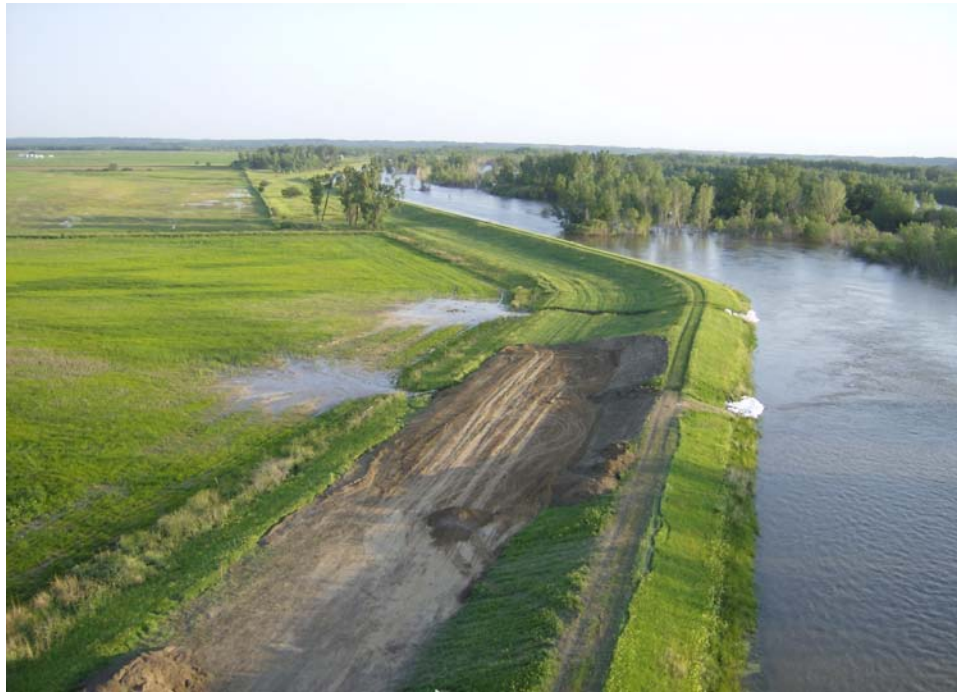
Figure 5. The levees along the Missouri River were subjected to prolonged water loading. Consequently, many suffered from erosion and underseepage, necessitating extensive repairs. (Photo taken June 2011 of levee L575 near Hamburg, Iowa.)
