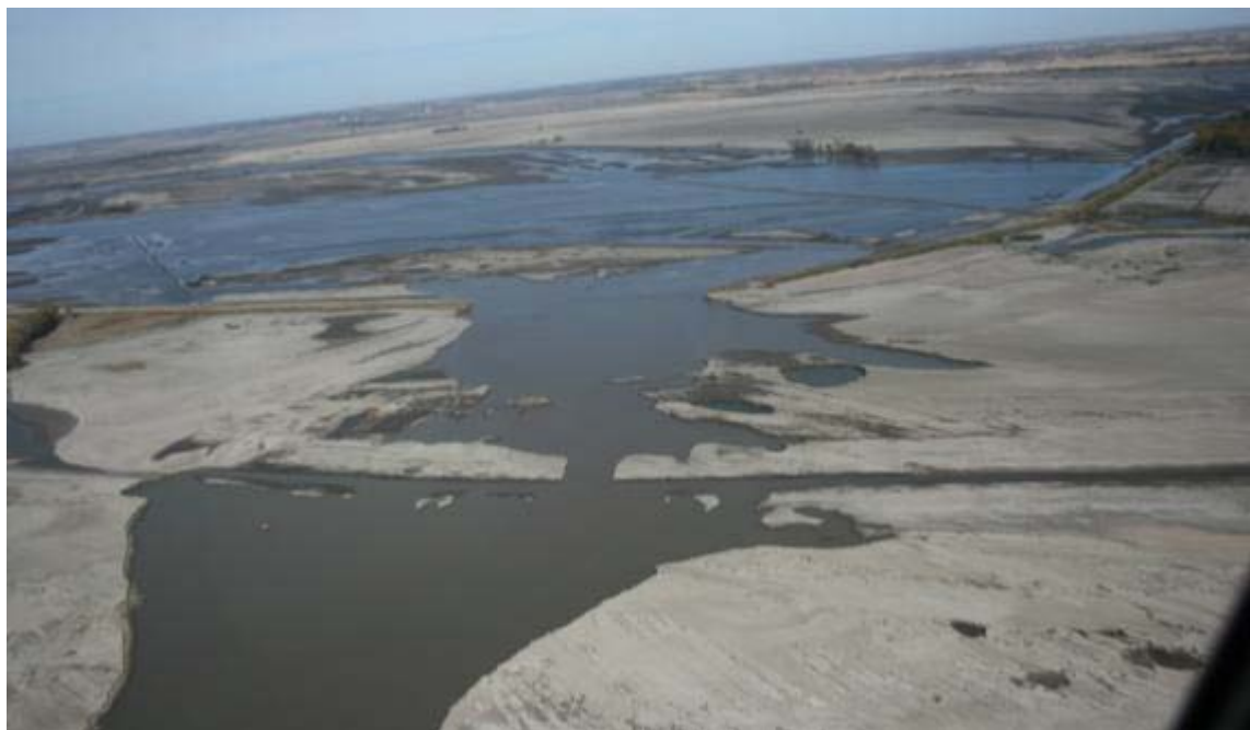
Figure 110. Levee breach: Lower breach at L575
