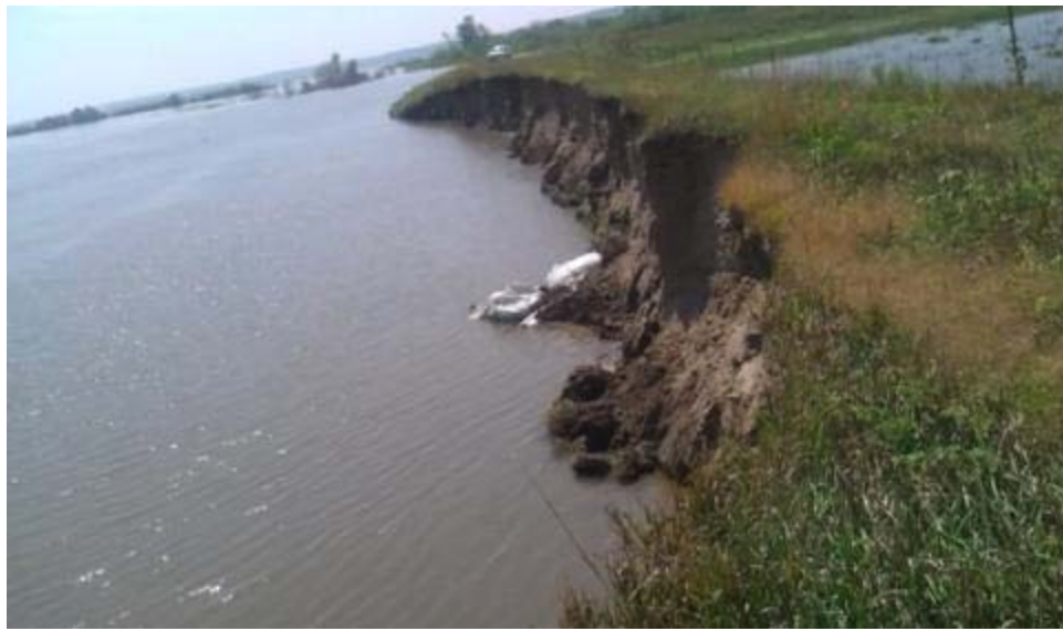
Figure 113. Levee scouring/erosion: L536 - Levee erosion – more than 50 percent of the embankment is missing – at MR Levee L536
