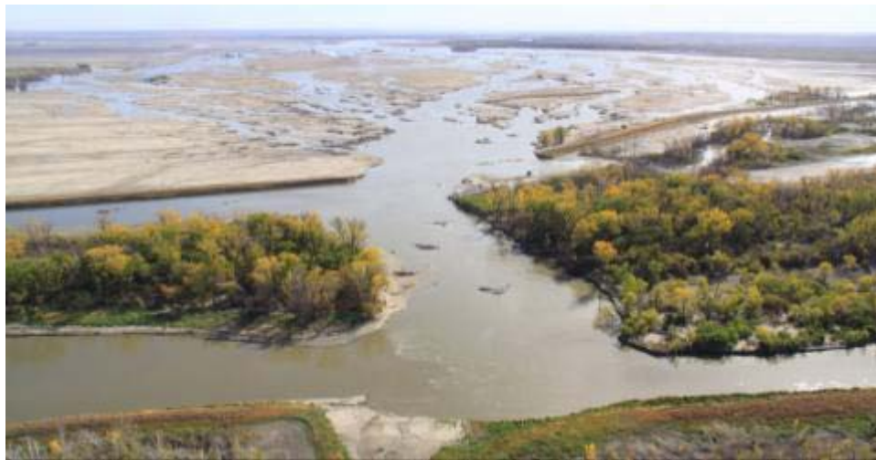
Figure 106. Levee breach: Middle breach at L575
