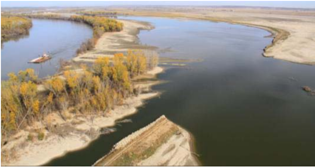
Figure 104. Levee breach: Upper breach at L575
