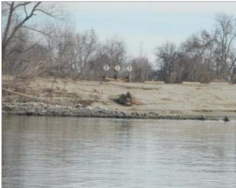
Figure 31. Dike Near River Mile 640.2
