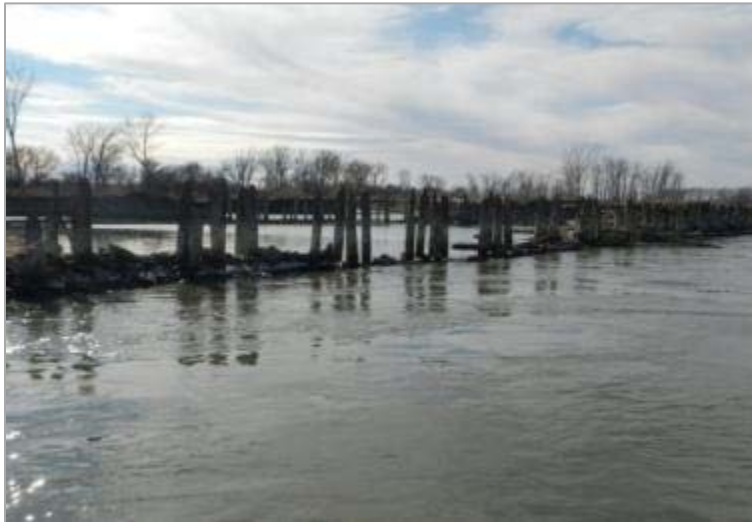
Figure 30. Revetment Near River Mile 679.8
