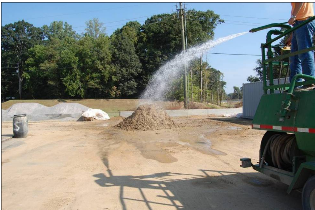
Figure 5. Hydro-seeder used to wet the soils.
