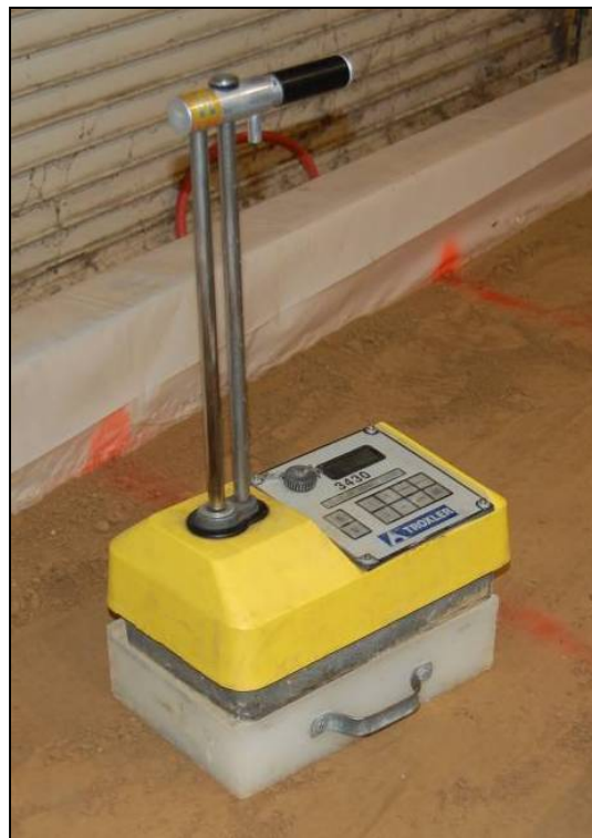
Figure 1. Nuclear moisture-density gauge used for testing.
