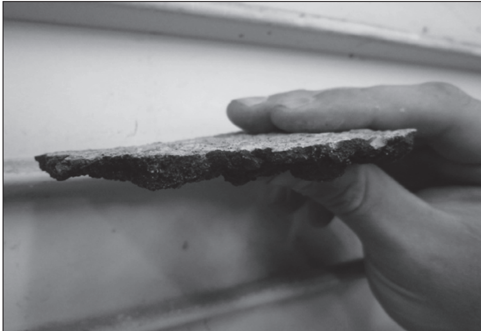
Figure 81. Asphalt material from oxidation test.
