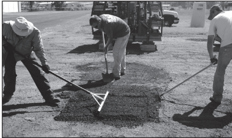
Figure A14. Preparing final lift for compaction.
