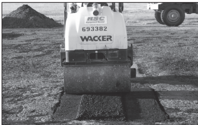
Figure A15. Compaction of final lift.
