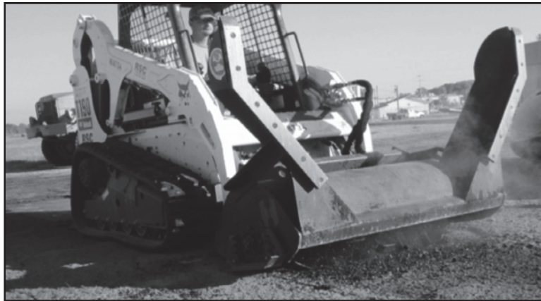
Figure A3. CTL-mounted asphalt processor.
