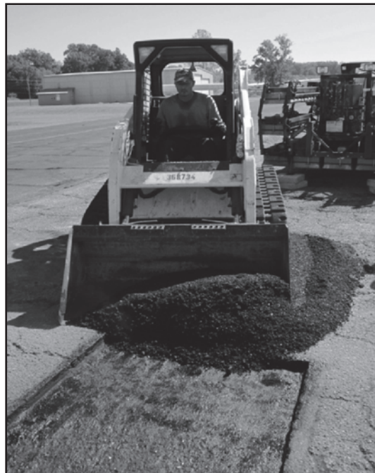
Figure 49. Rejuvenated stockpile being placed into repair void.
