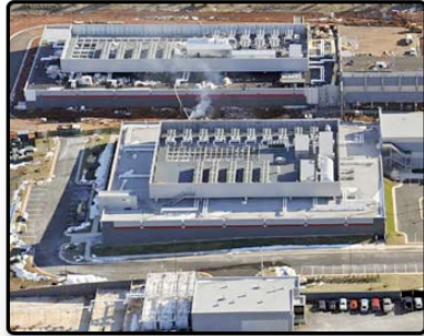
Terremark Data Center
