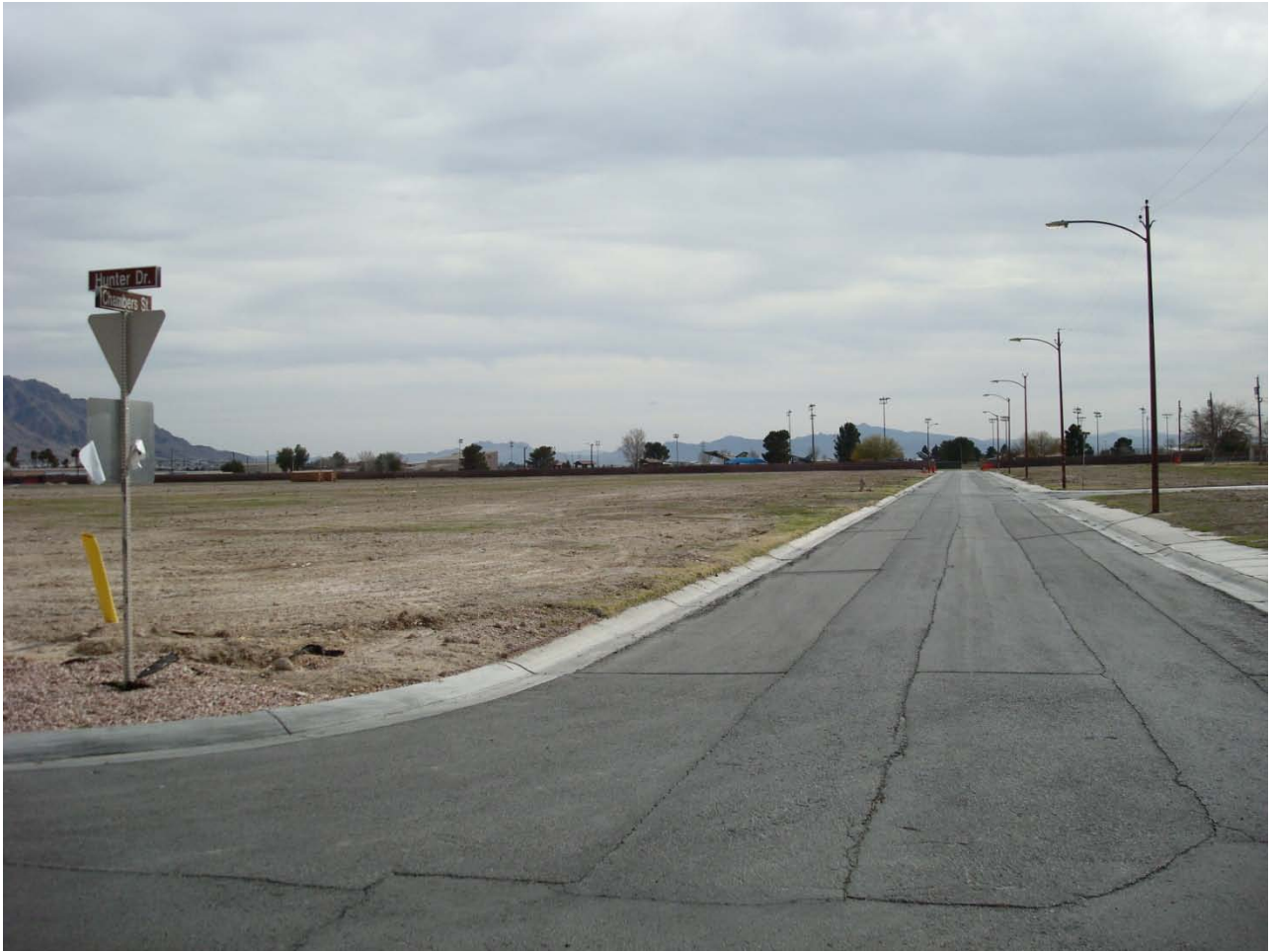
Figure 7-a. Parcel E-1 western boundary Chambers St. looking south
