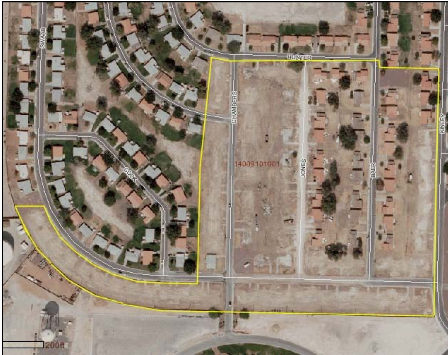
Figure 6. Aerial photo of Parcel E-1 taken in 2009 during housing demolition.
