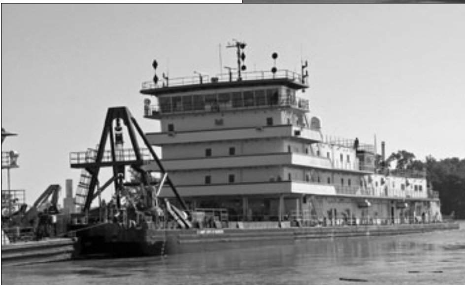
Below: Dredge Hurley, Memphis District
