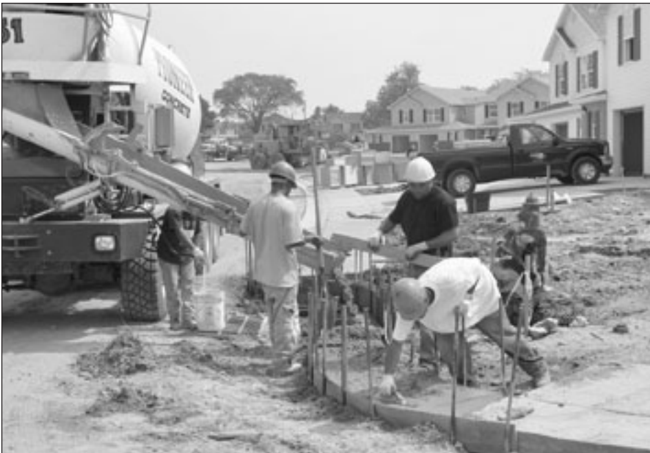
Building new family housing units at Dover Air Force Base
