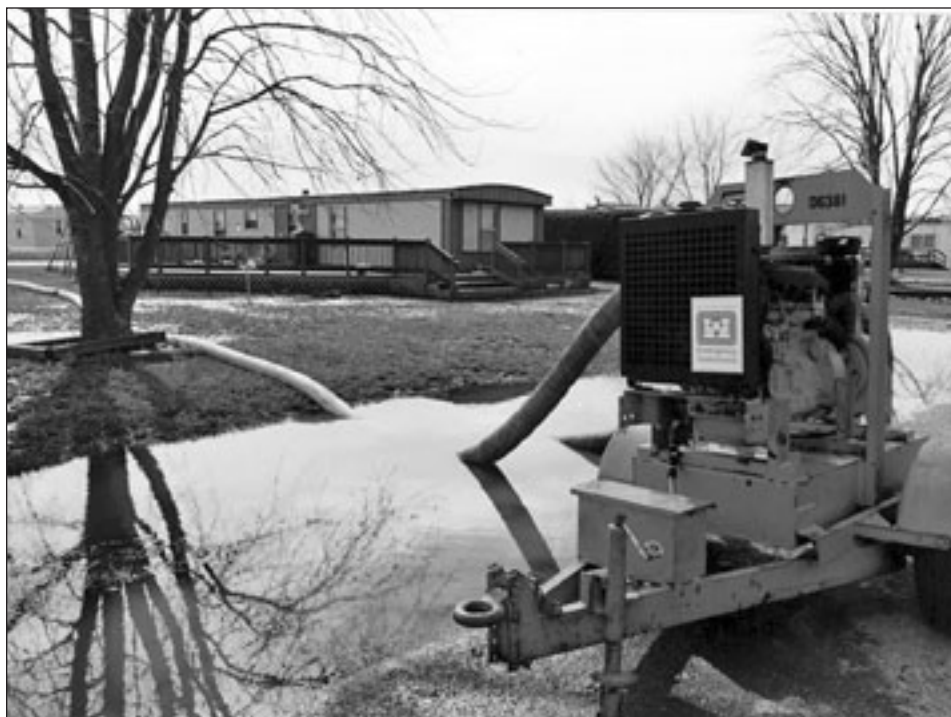
Emergency equipment on loan from the Philadelphia District pumps down flood waters in Sussex County, Del.
