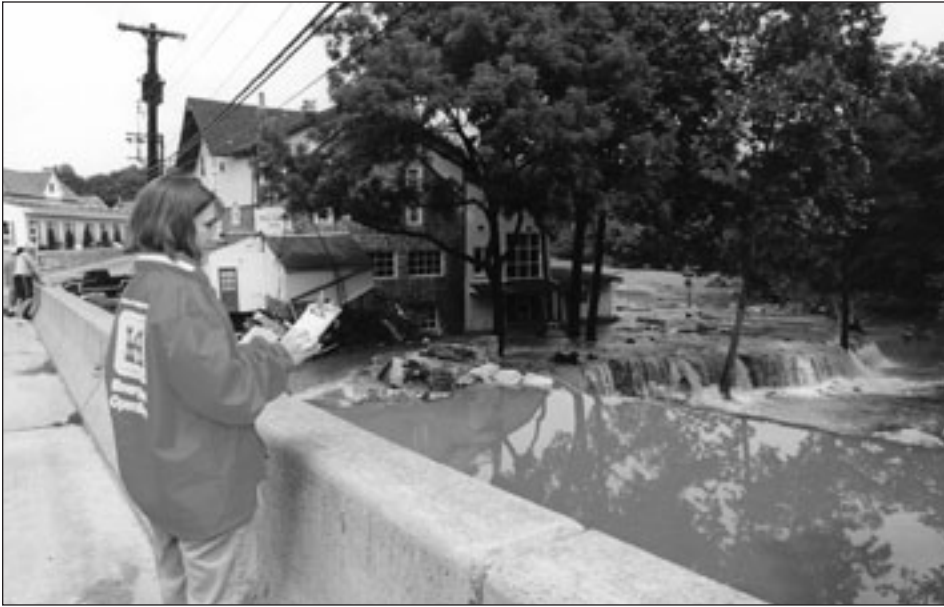
Philadelphia District personnel conducting flood damage surveys in Bucks County, Pa.
