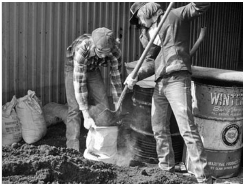
Filling sandbags for flood-fighting
