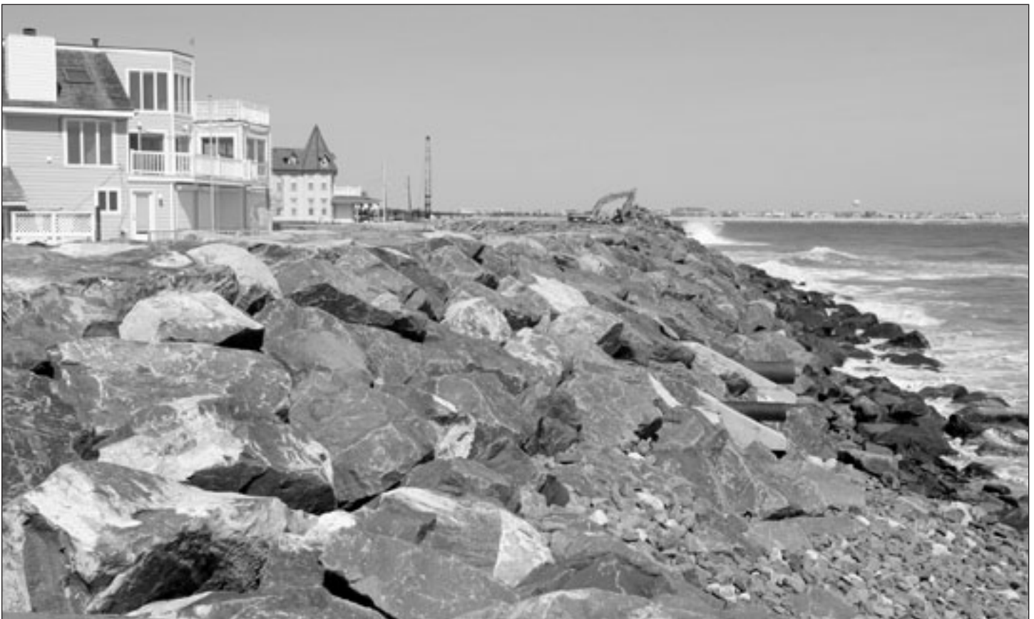
The seawall at Avalon, N.J., upgraded by the district as part of the Townsends Inlet to Cape May Inlet Coastal Storm Damage Reduction Project
