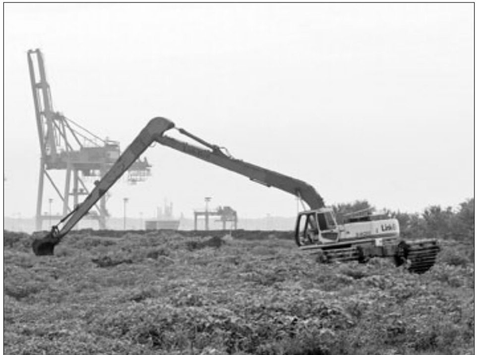
The Wilmington Harbor South confined disposal facility
