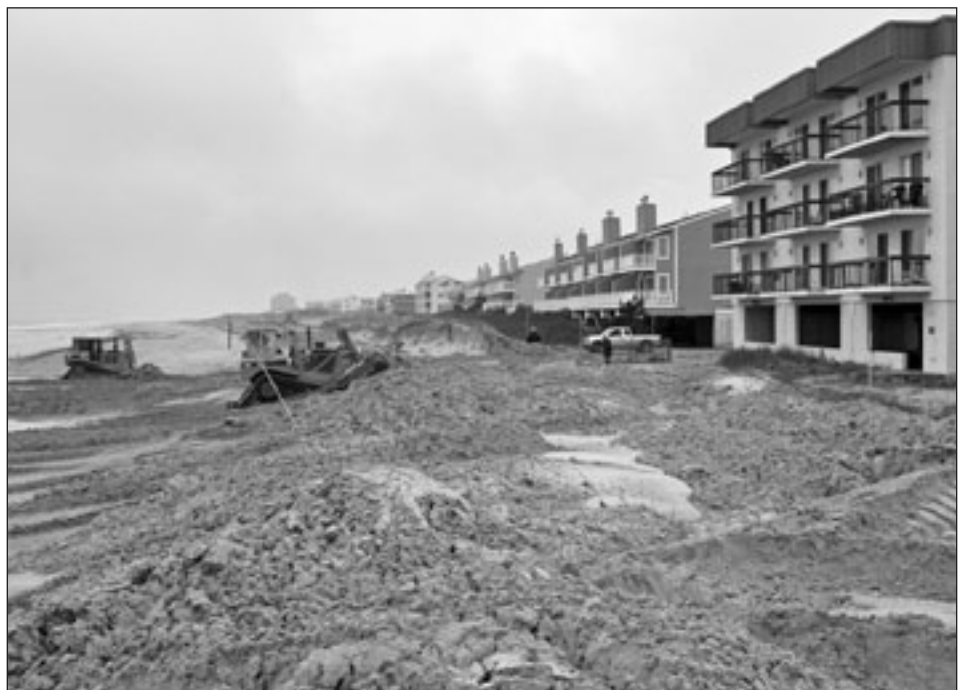
Initial beach nourishment at Brigantine, N.J.
