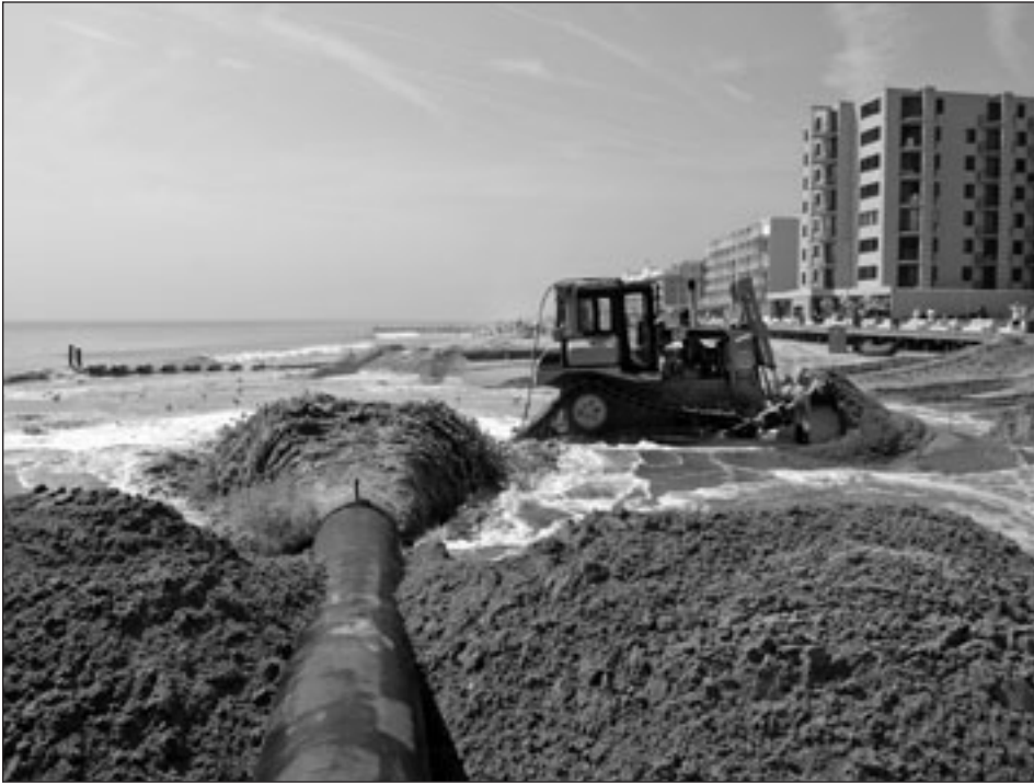
Beachfill operations at Rehoboth Beach, Del.
