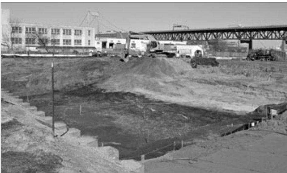
Cleanup of the Welsbach & General Gas Mantle site in and near Camden, N.J., involved a multi-year, multi-phase project to remove radiological contamination
