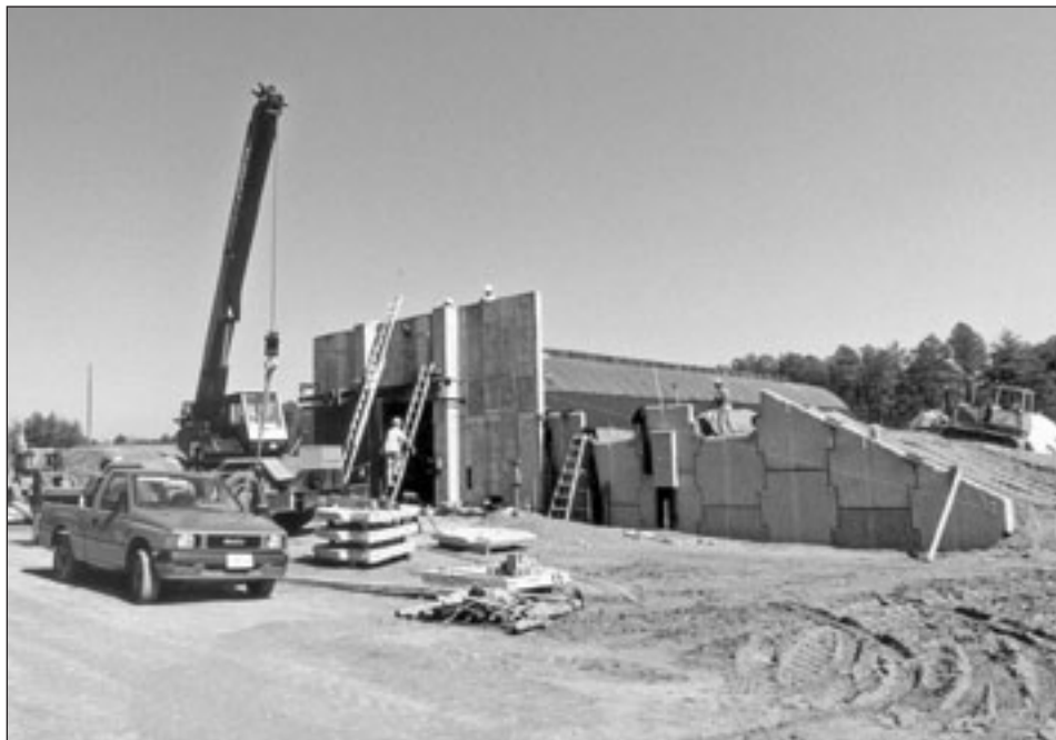
Fort Dix ammunition storage facility under construction
