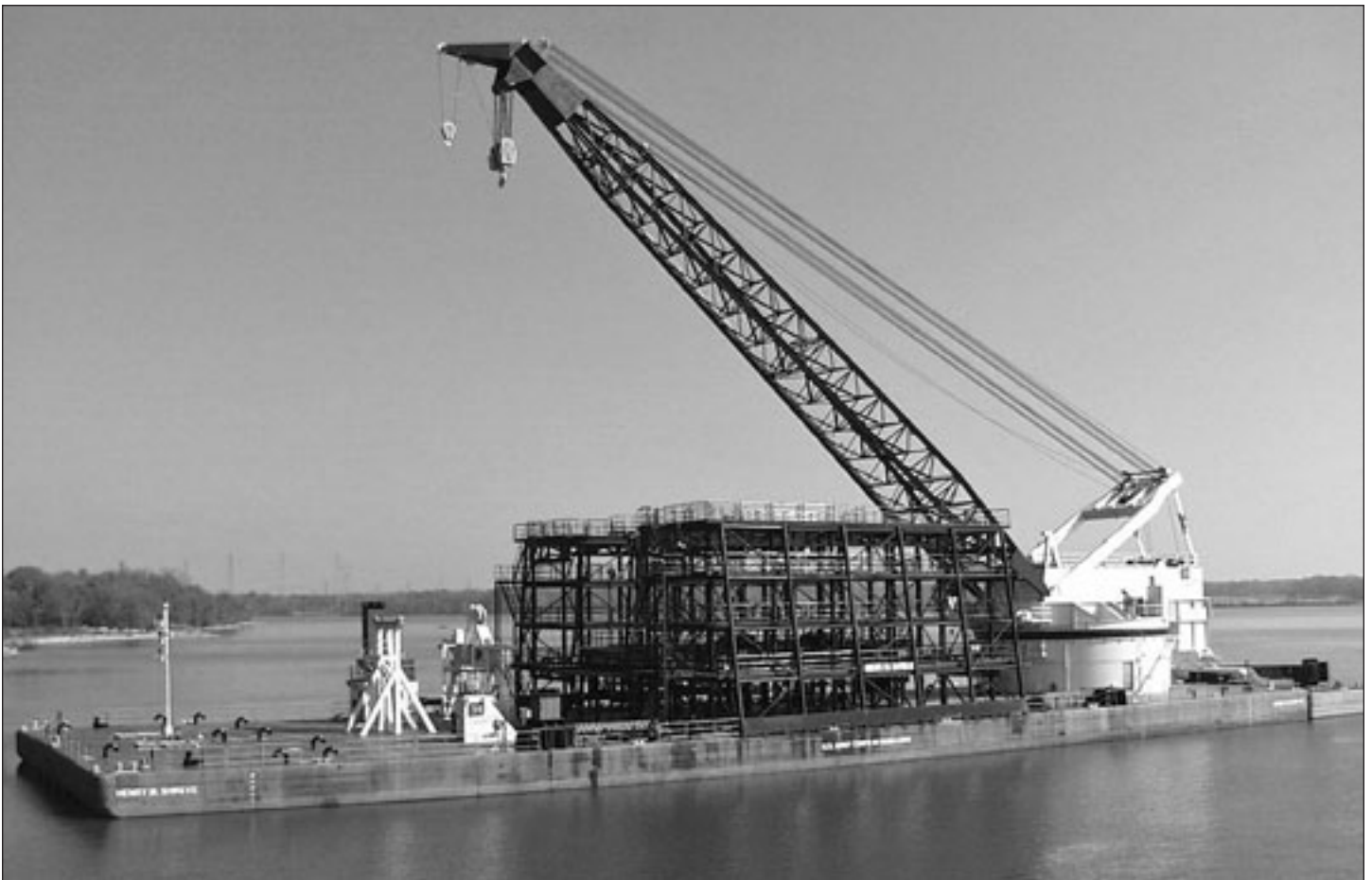
Crane Barge Henry M. Shreve
