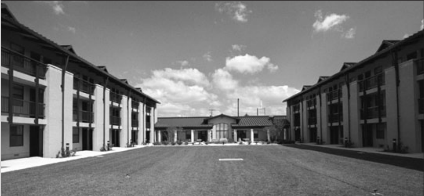
Airman dormitories at Dover
