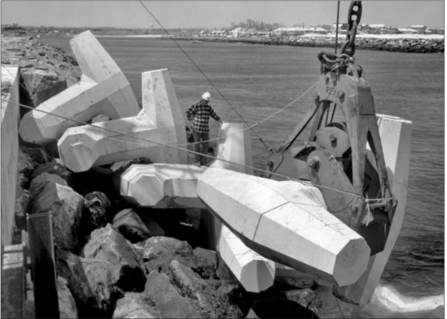
Putting the dolosse into place at Manasquan Inlet
