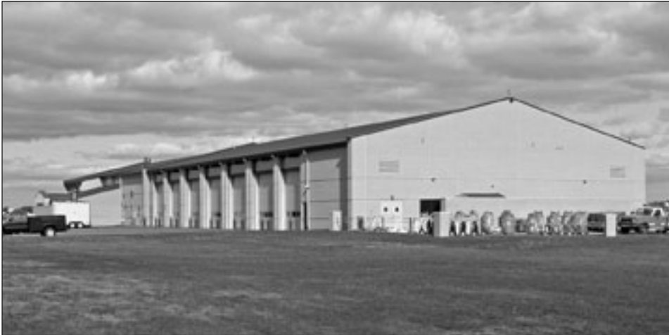
Fire/Crash Rescue Station, Dover Air Force Base
