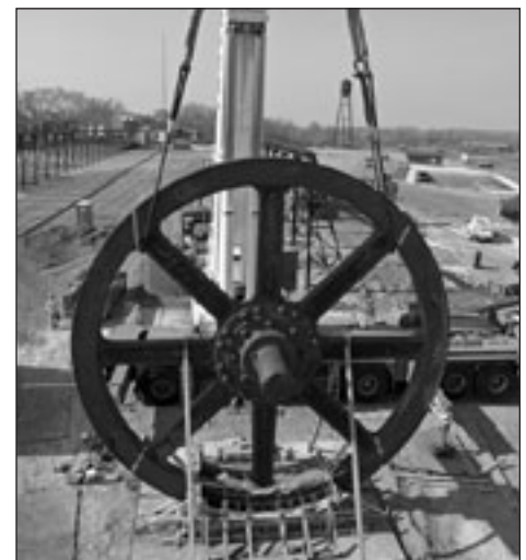
Remediation of the Roebling Steel Company Superfund site involved preservation and restoration of historic artifacts, such as the old gatehouse and this 124-ton, 28-foot-diameter flywheel, both now part of the Roebling Museum
