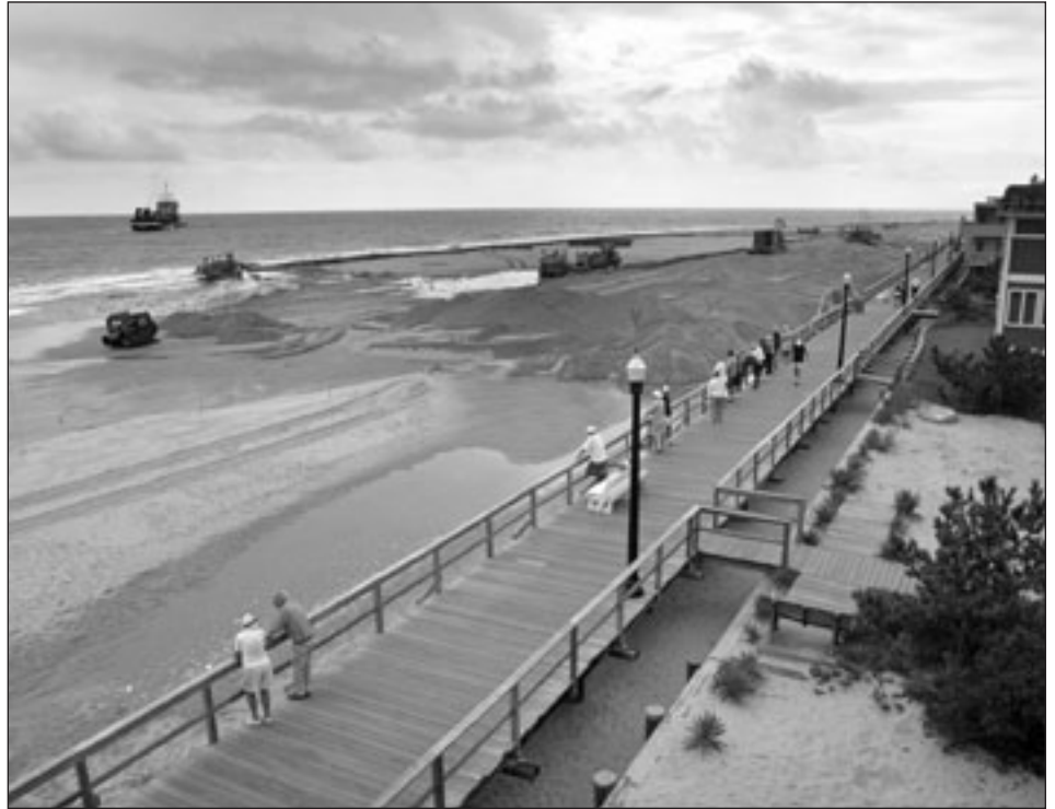
Construction of the Bethany Beach/ South Bethany Project
