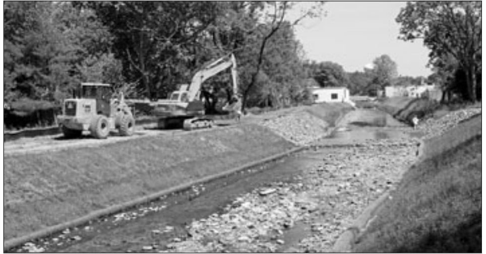
Construction of the Little Mill Creek Flood Control Project in Delaware
