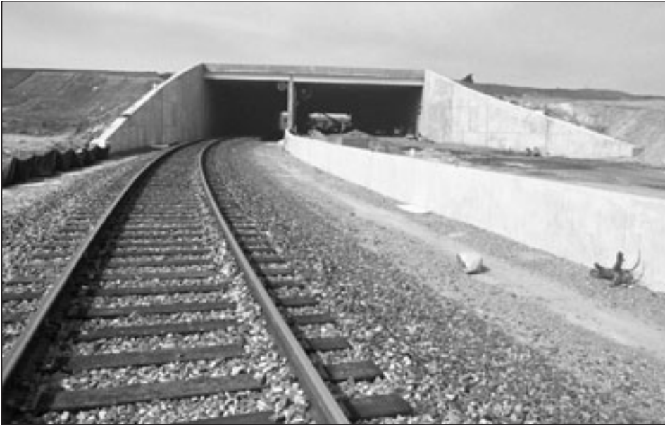
The Philadelphia International Airport Runway Project under construction
