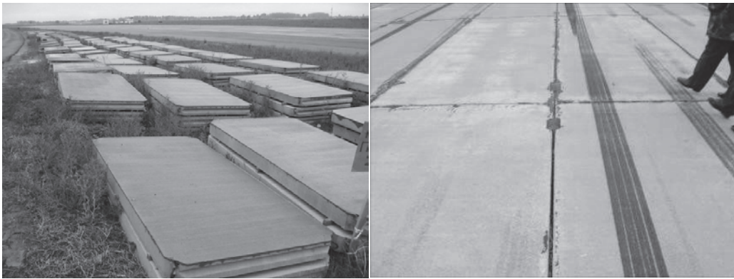
Figure 2. (left) Stockpiled precast panels at a Soviet airfield and (right) precast concrete panel runway still in service (Tingle et al. 2007).
