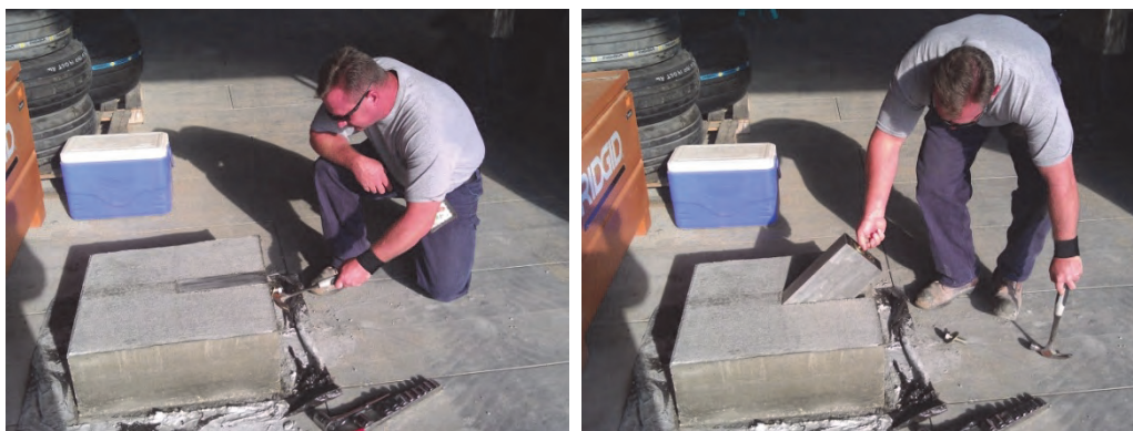
Figure A13. Removing the steel blockouts.
