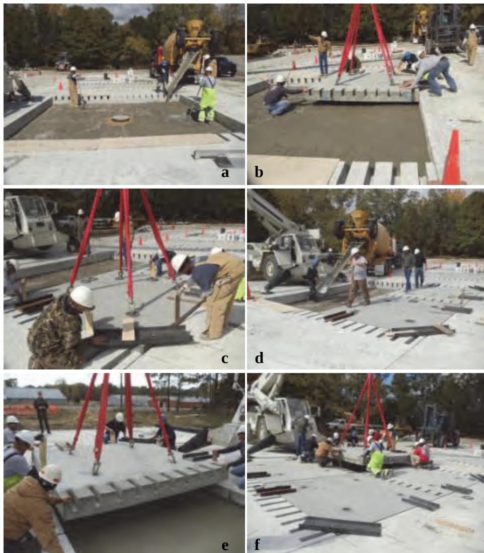
Figure 58. Installation of Repair 3 panels: a) pedestal location; b) placing first panel; c) using shims to place second panel; d) placing flowable fill for third and fourth panels; e) placing third panel; f) placing fourth panel.
