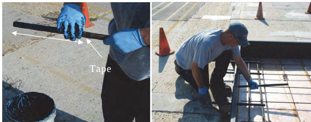
Figure A8. Installation of dowels.
