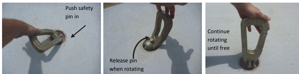
Figure B20. Removing swift lifting eyes.
