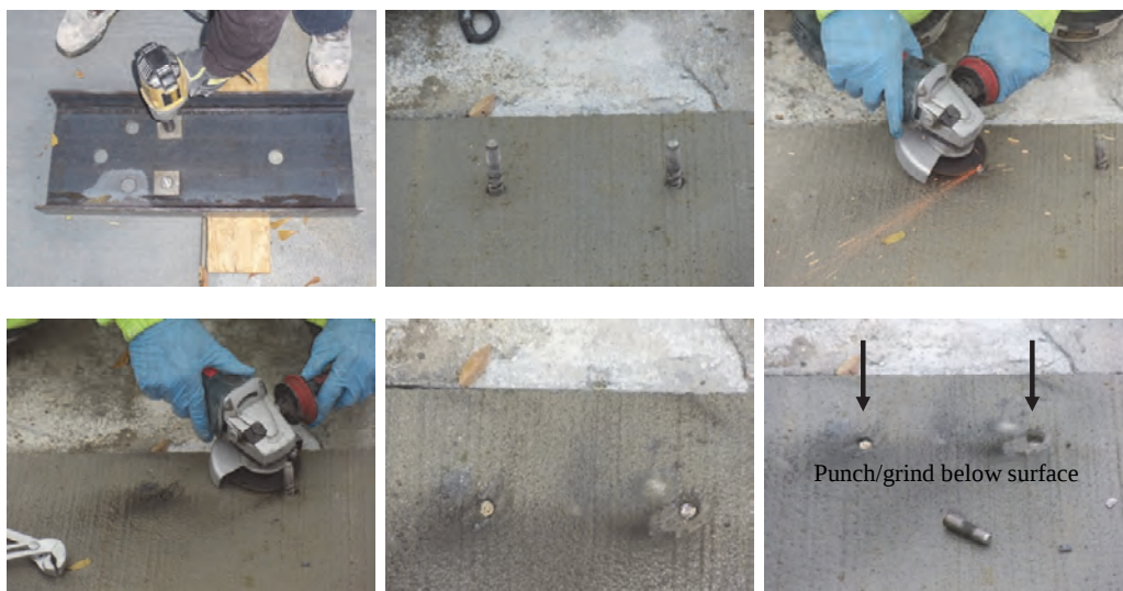
Figure B22. Bridge plate removal.
