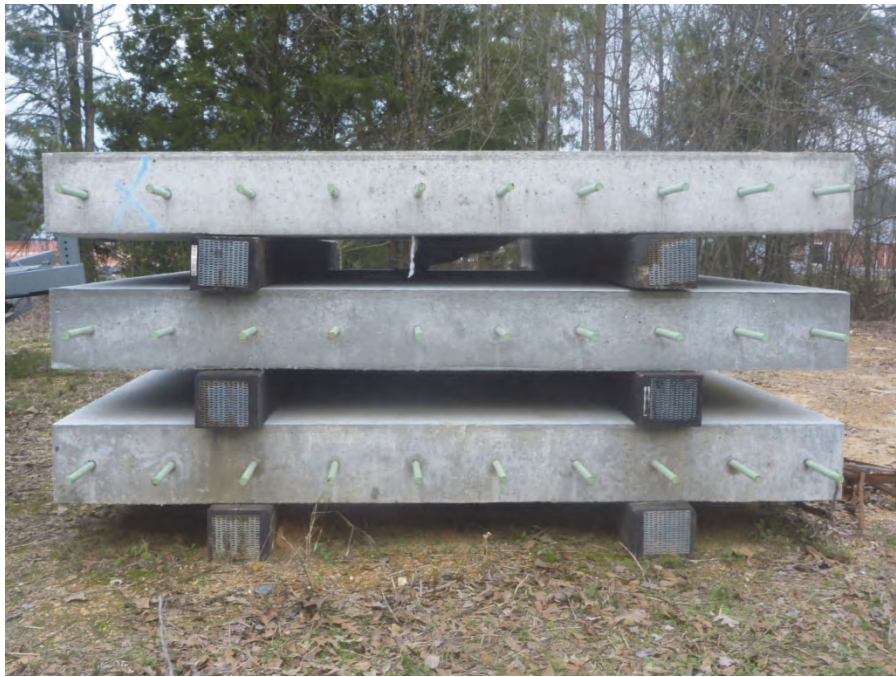
Figure 34. Panels stacked on dunnage.
