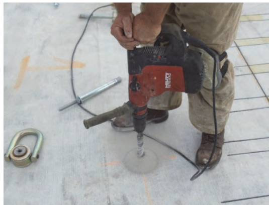
Figure B4. Drilling expansion anchor hole.
