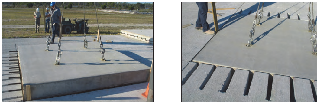
Figure 4. Air Force method installation (Ashtiani et al. 2010).
