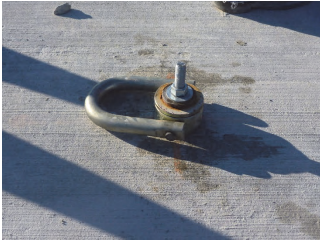
Figure B6. Installed expansion anchor and swivel hoist ring prior to tightening.
