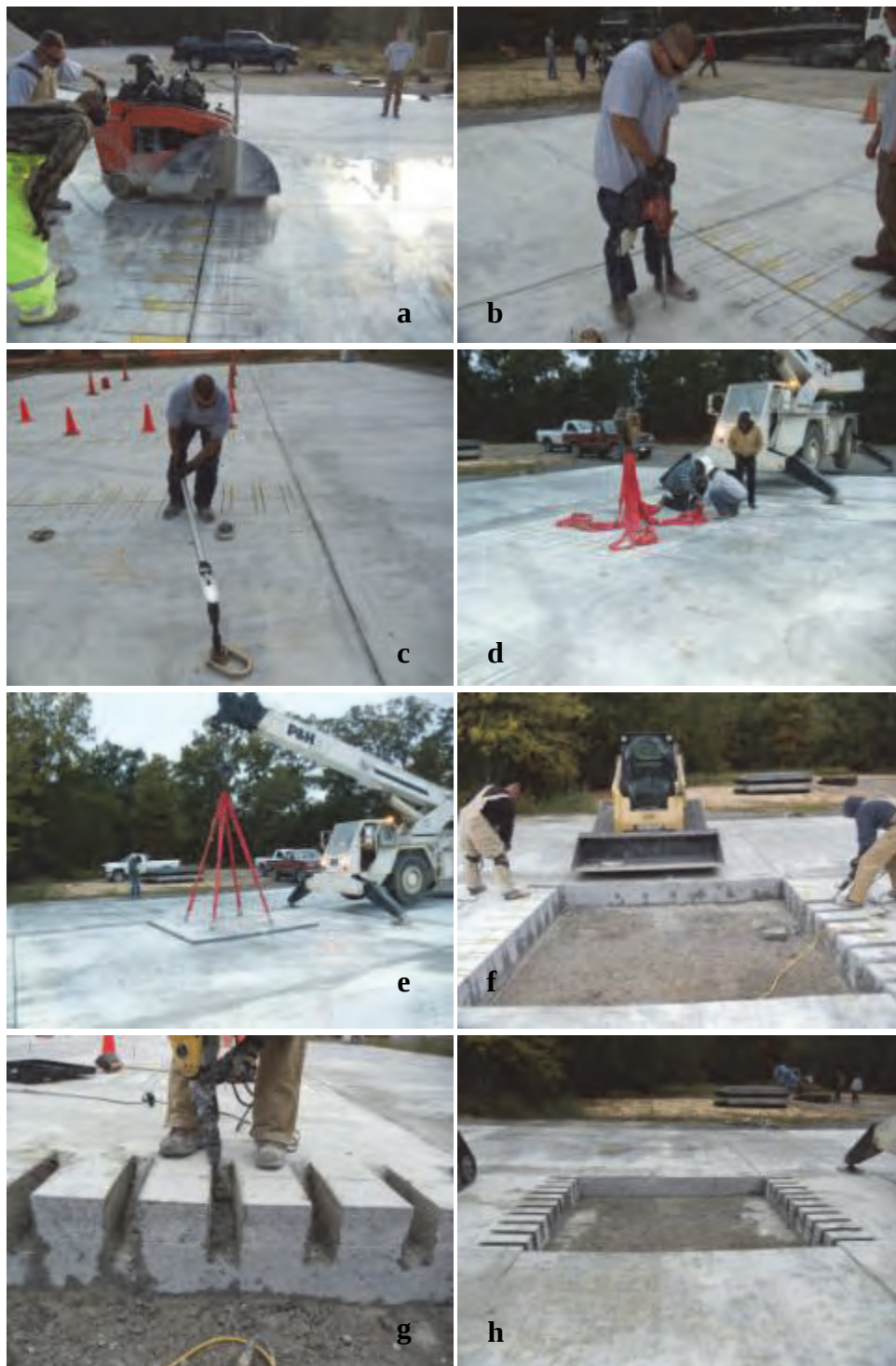
Figure 52. Preparation and removal of parent PCC: a) saw cutting dowel receptacles and repair area; b) drilling to install concrete lifting anchors; c) installing lifting eyes; d) connecting lifting eyes to crane rigging; e) lifting “damaged” pavement; f) preparation of dowel receptacles using jackhammers; g) close up of dowel receptacles; and h) prepared repair area.
