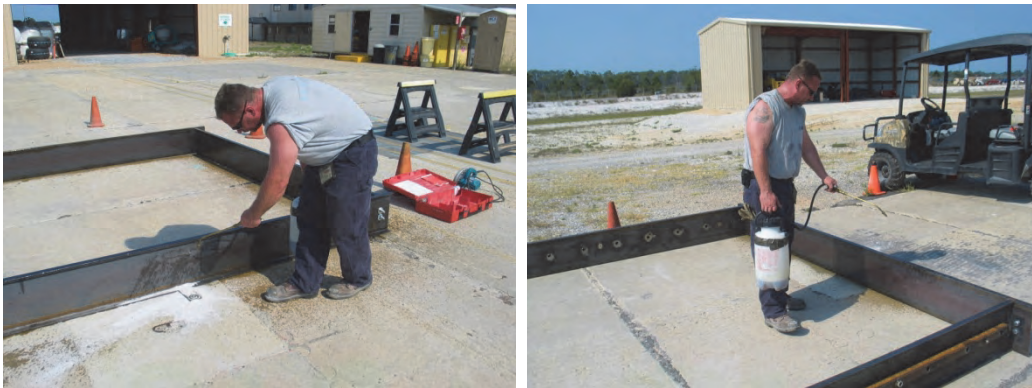
Figure A5. Application of release agent.
