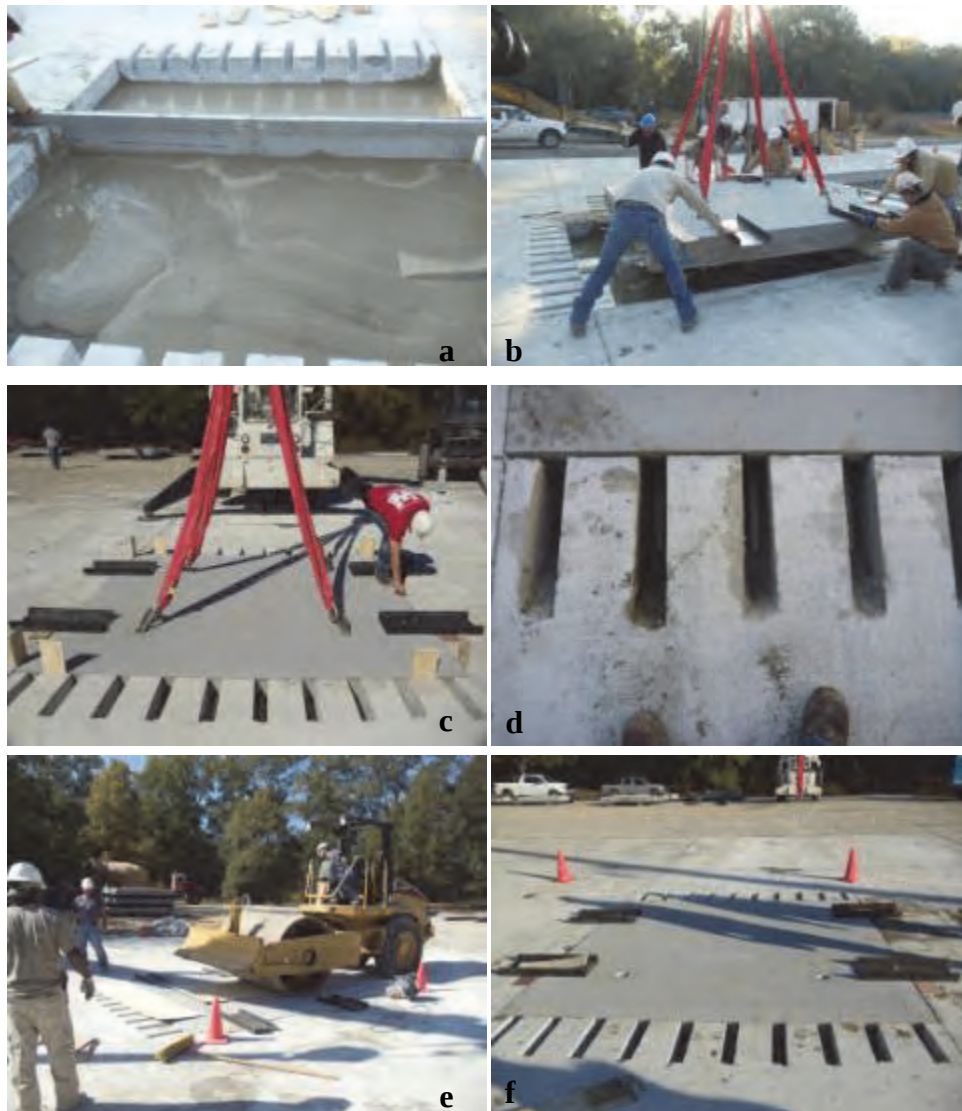
Figure 55. Placement of precast panel: a) screeding of flowable fill; b) placing panel; c) placed panel with plywood spacers; d) close up of dowels in dowel receptacles; e) using compactor to seat panel; and f) panel prior to dowel receptacle grouting.
