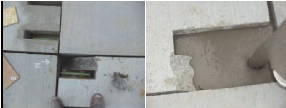
Figure 59. Left: broken corner of a panel, and Right: repair of broken corner.
