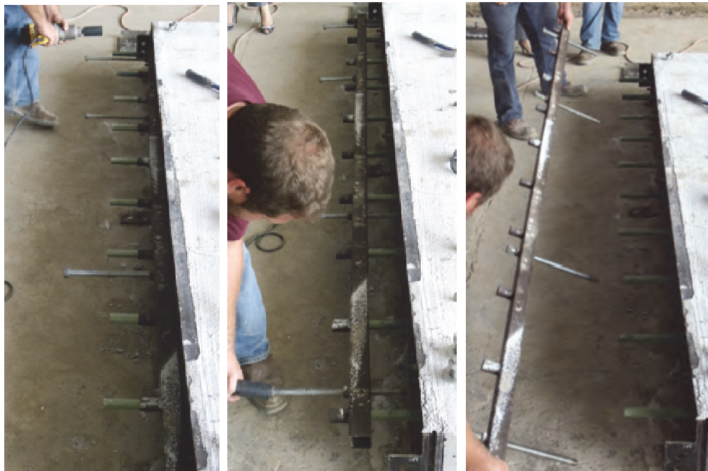
Figure 19. Removal of dowel bar holder.
