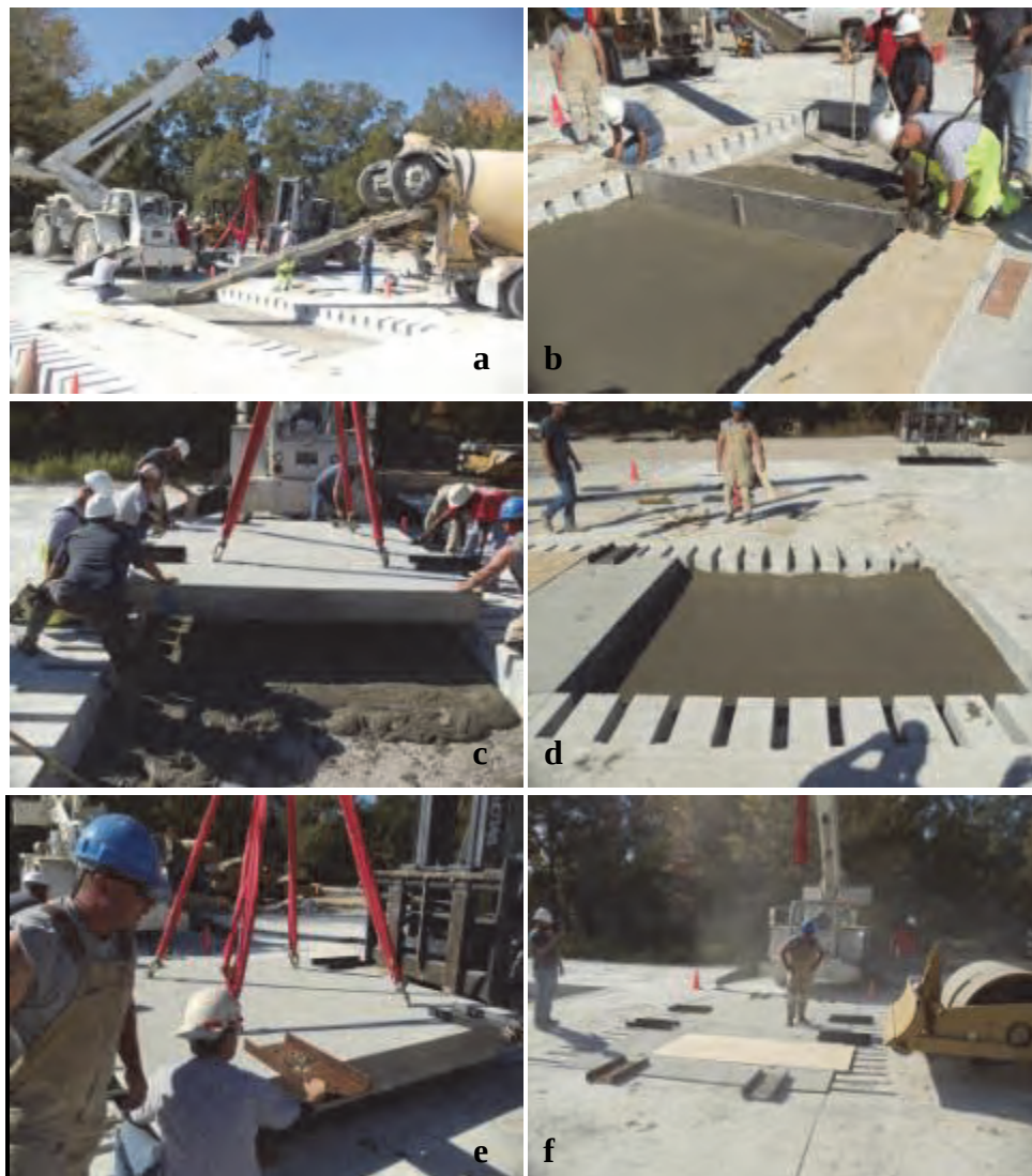
Figure 57. Placement of two panels in Repair 2: a) placing flowable fill and reading first panel; b) screeding flowable fill for first panel; c) placing first panel; d) placed flowable fill for second panel; e) placing second panel; f) seating panel using roller compactor.
