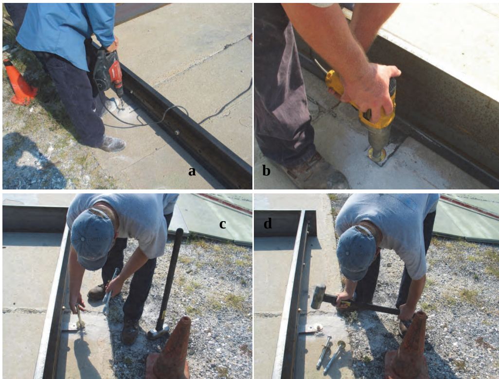
Figure A4. Anchoring the formwork.
