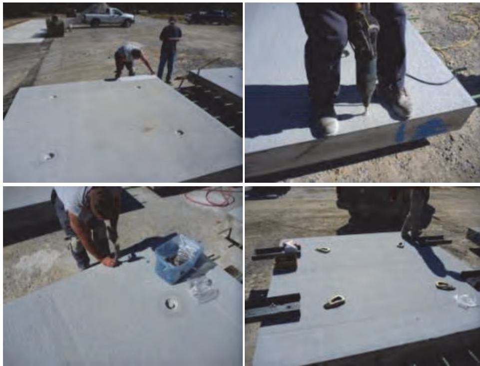
Figure 54. Installation of bridge plates: clockwise from top left: using template to mark anchor locations, drilling holes for anchors, installing anchor, and completed bridge plate installation and lifting eyes.
