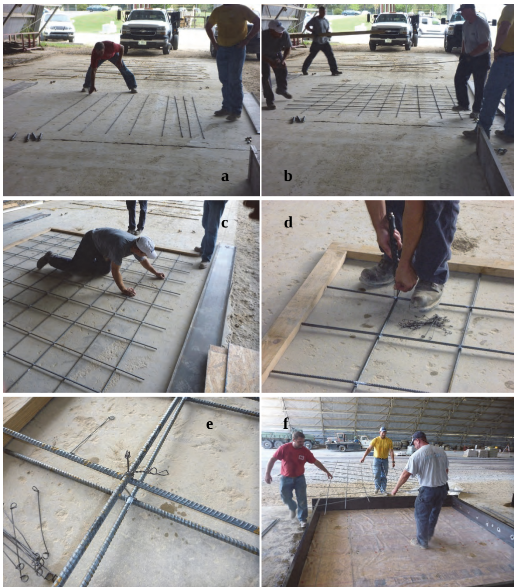
Figure A6. Constructing the rebar grid.
