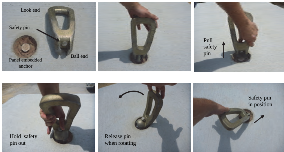
Figure A15. Installing lifting eyes.
