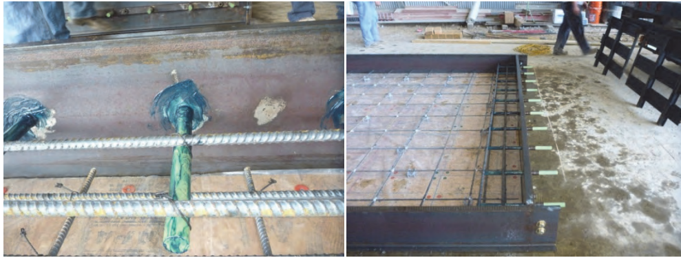
Figure A9. Locations of #5 rebar.
