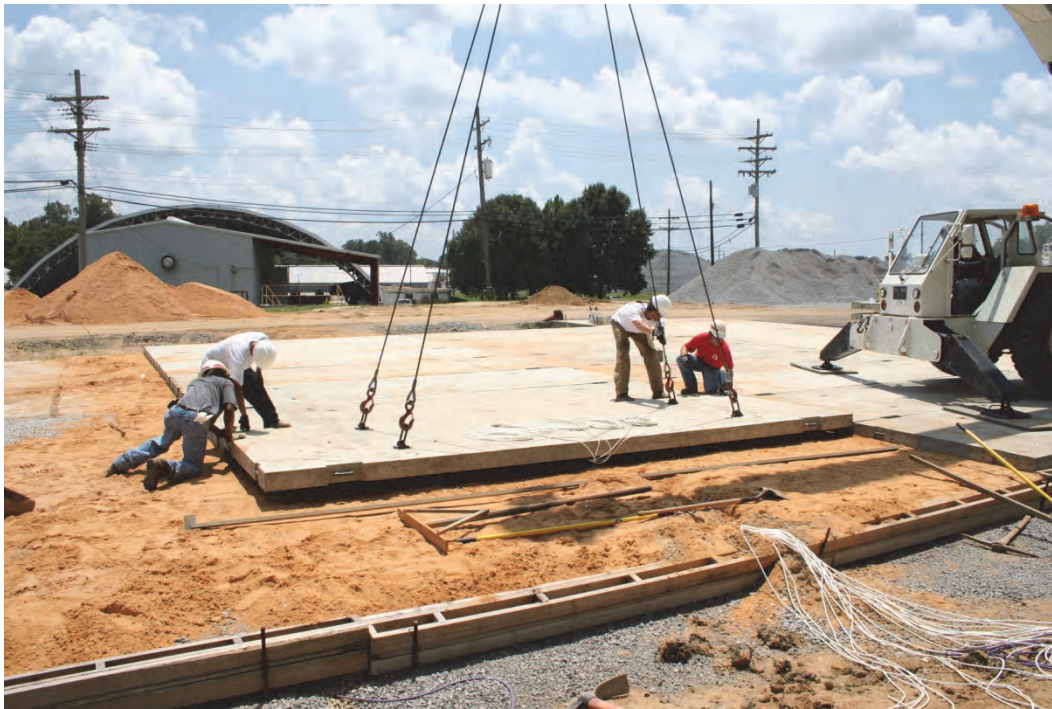
Figure 3. Placement of a precast panel (Tingle et al. 2007).
