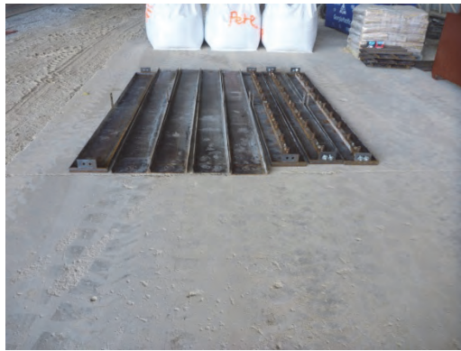
Figure A2. Organized formwork.
