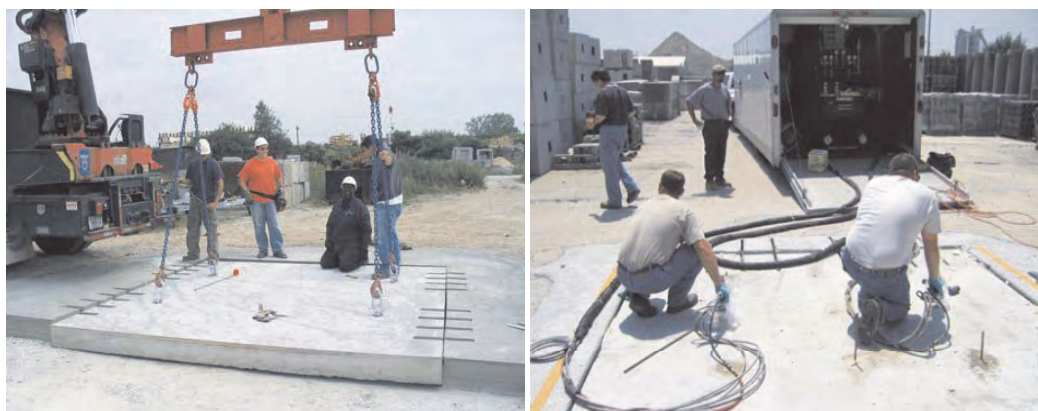
Figure 9. (Left) installing Roman Road slab; (right) injecting polyurethane foam (Roman Stone Co. 2012).
