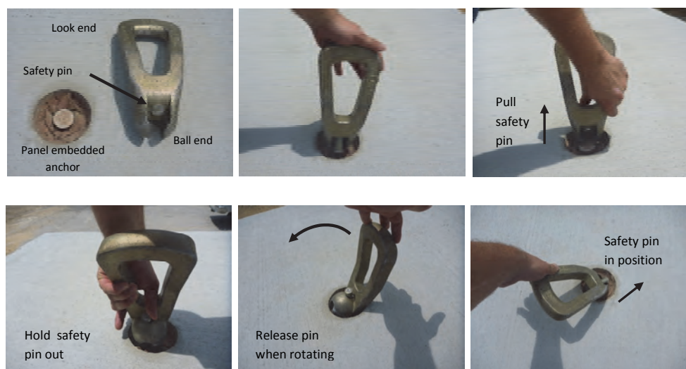
Figure B16. Attaching lifting eyes to embedded panel anchors.
