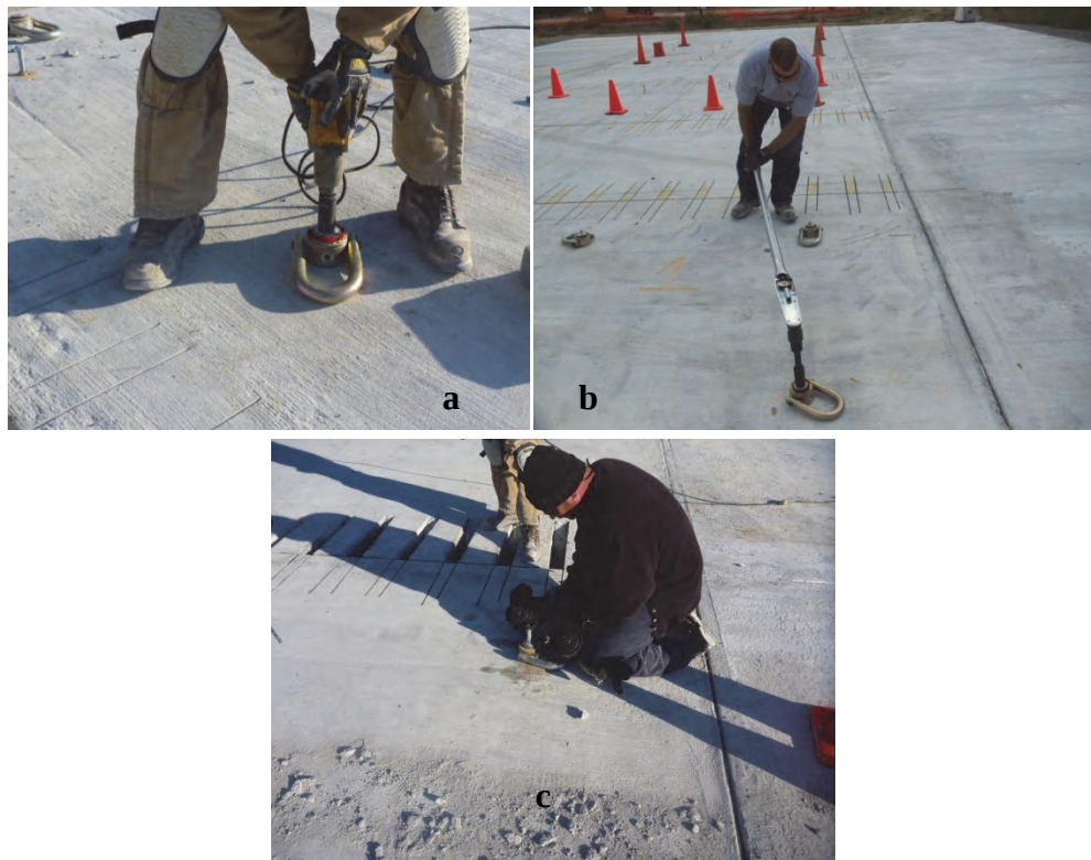
Figure B7. Activating the expansion anchor.
