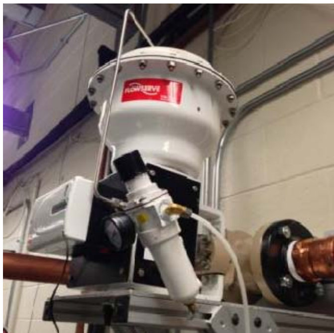
Figure D.6: 3" air line mass flow controller
