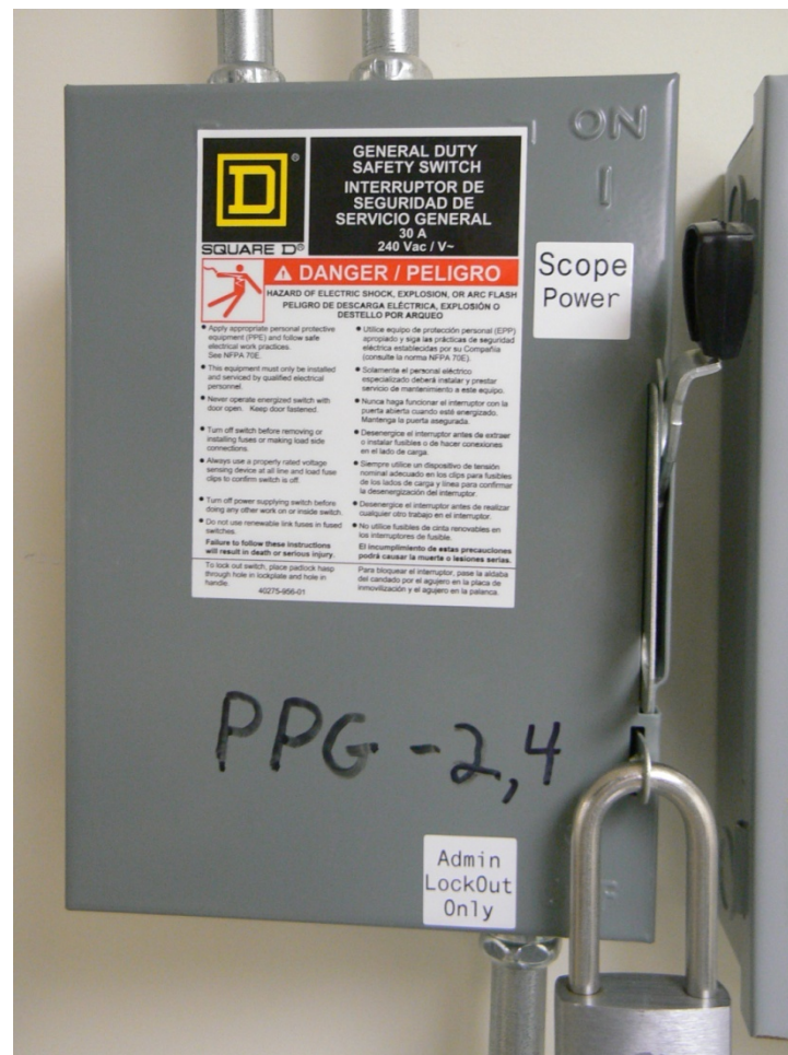
Figure 13. General Duty Safety Switch with Administrative Lock
