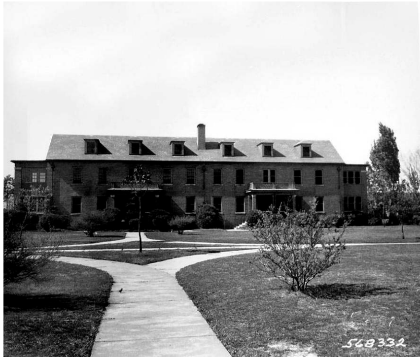
Figure 247: Student Apartments (NARA 165-FF Box 9B, 20-21).
