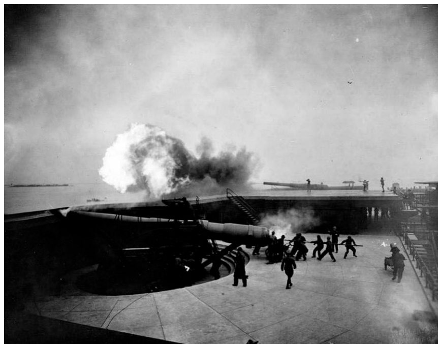
Figure 304: Guns on Battery, 1918 (NARA RG 111-SC Box 451 55954).
