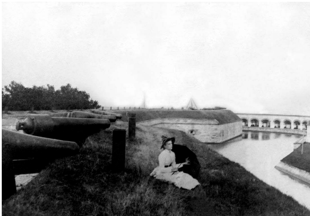
Figure 262: View from terreplein (NARA 165-FF Box 9B, 20-21).
