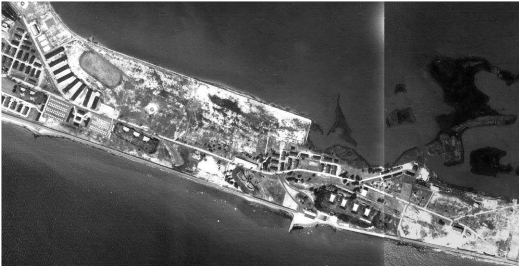
Figure 402: Aerial view, 1948 (Fort Monroe Cultural Resources).
