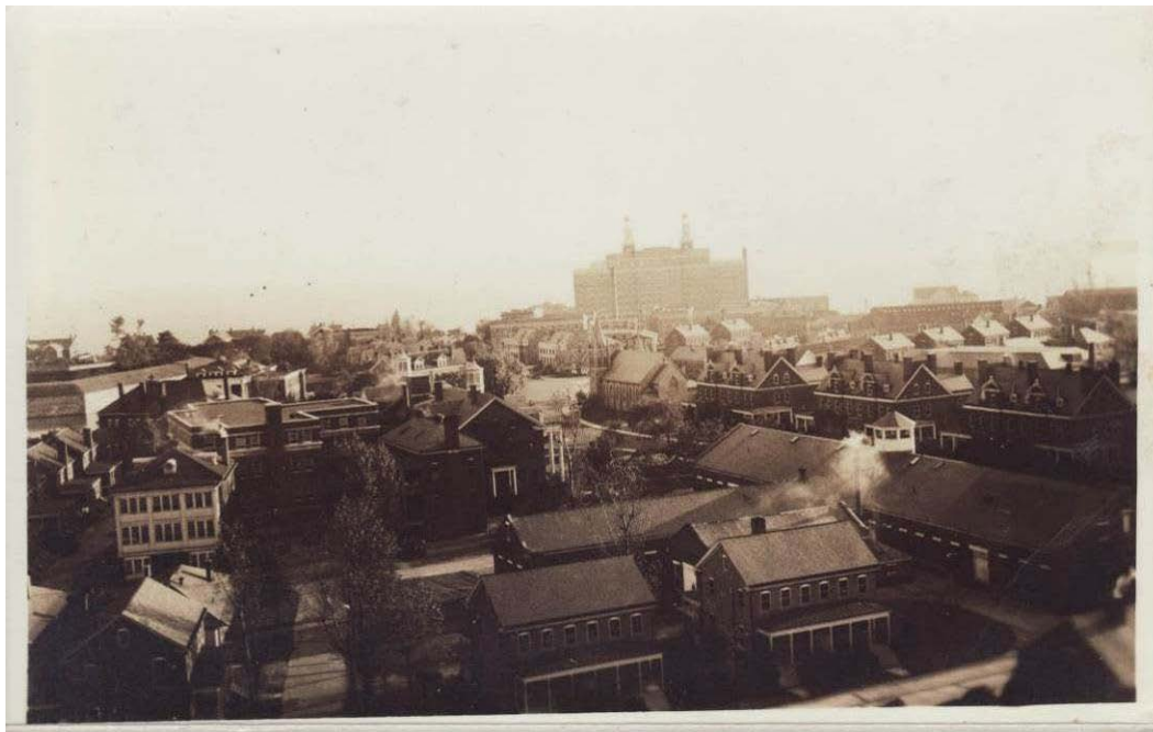
Figure 198: Post card view toward Hotel Chamberlin (Casemate Museum).
