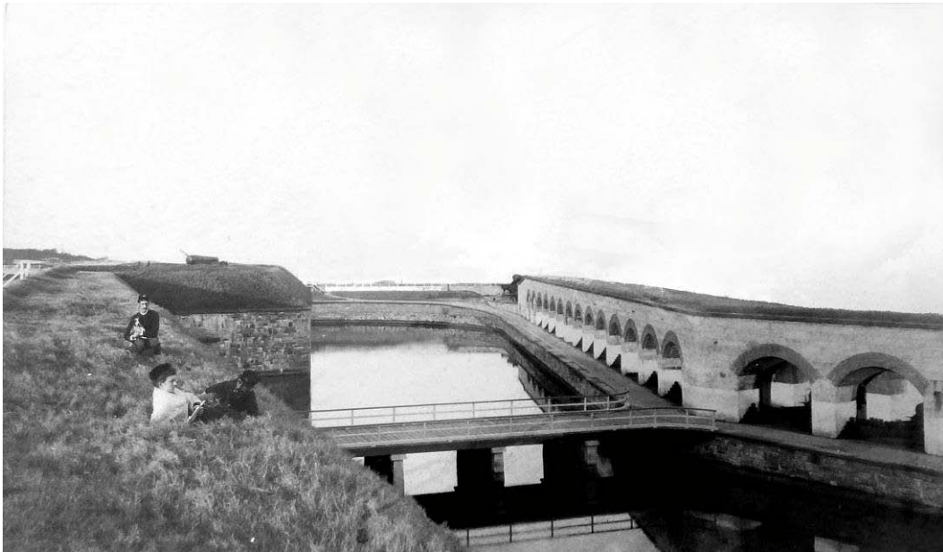
Figure 259: View of Water Battery (NARA 165-FF Box 9B, 20-21).
