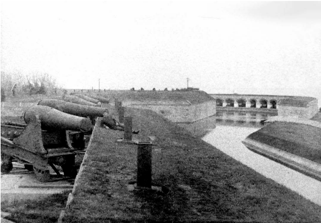
Figure 263: View from terreplein (NARA 165-FF Box 9B, 20-21).
