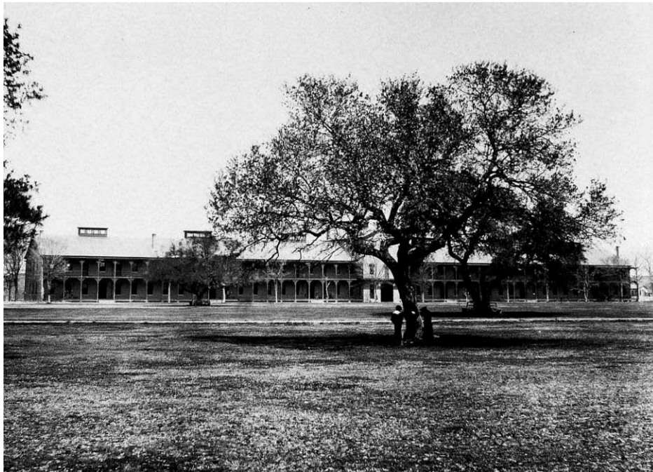
Figure 208: Barracks, Building 5 (NARA 165-FF Box 9B, 20-21).
