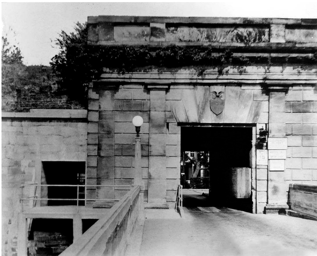
Figure 252: Main Gate (NARA 165-FF Box 9B, 20-21).
