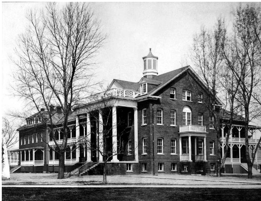
Figure 224: Post Hospital (NARA 165-FF Box 9B, 20-21).
