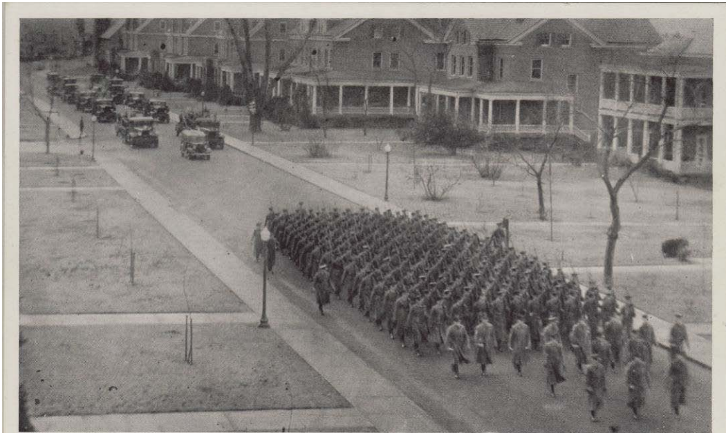
Figure 148: Post card of parade along Ingalls Road (Casemate Museum).
