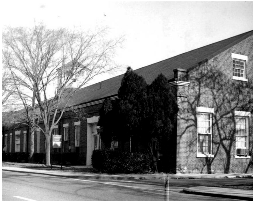
Figure 329: Building 27, 2 Mar 1971 (NARA CC 75163).
