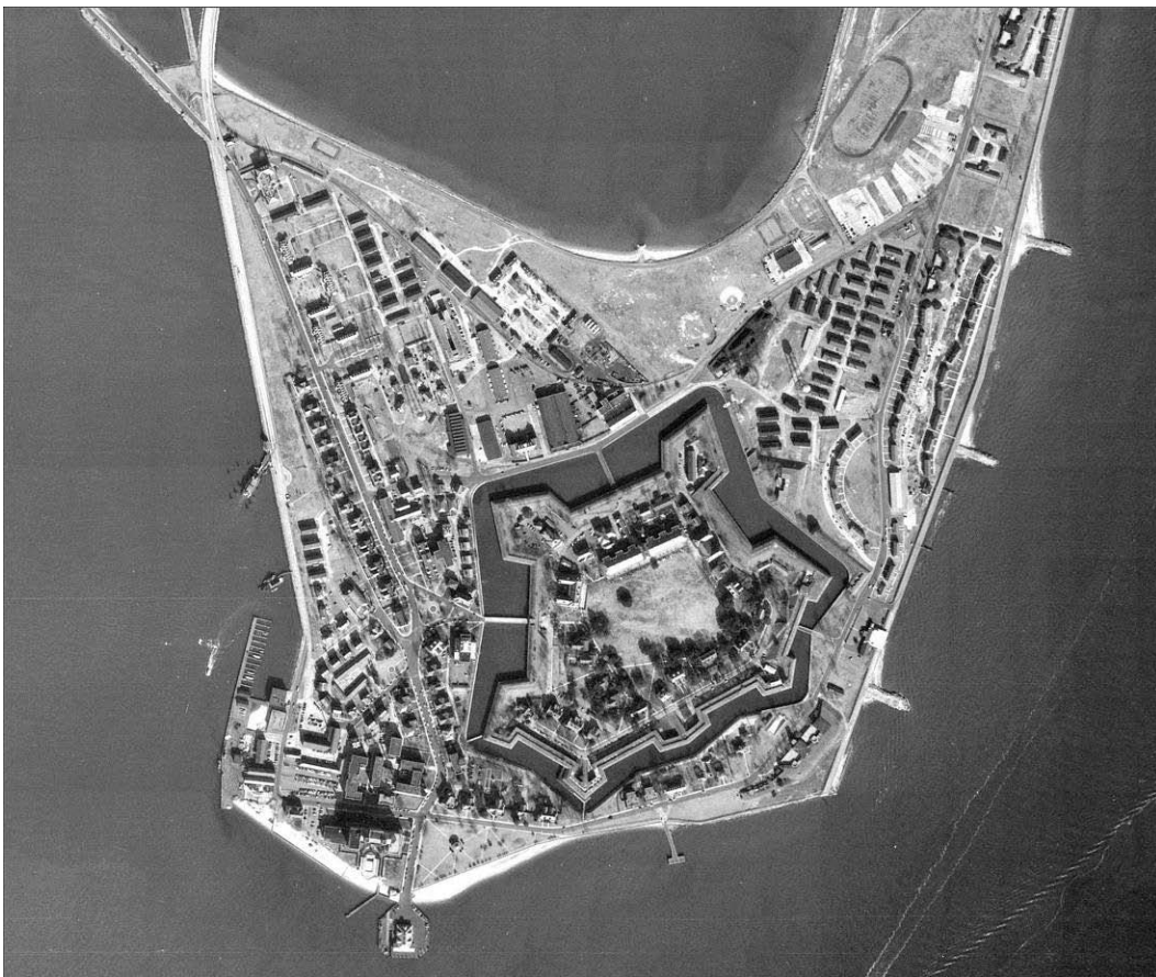
Figure 403: Aerial view, 1954 (Fort Monroe Cultural Resources).
