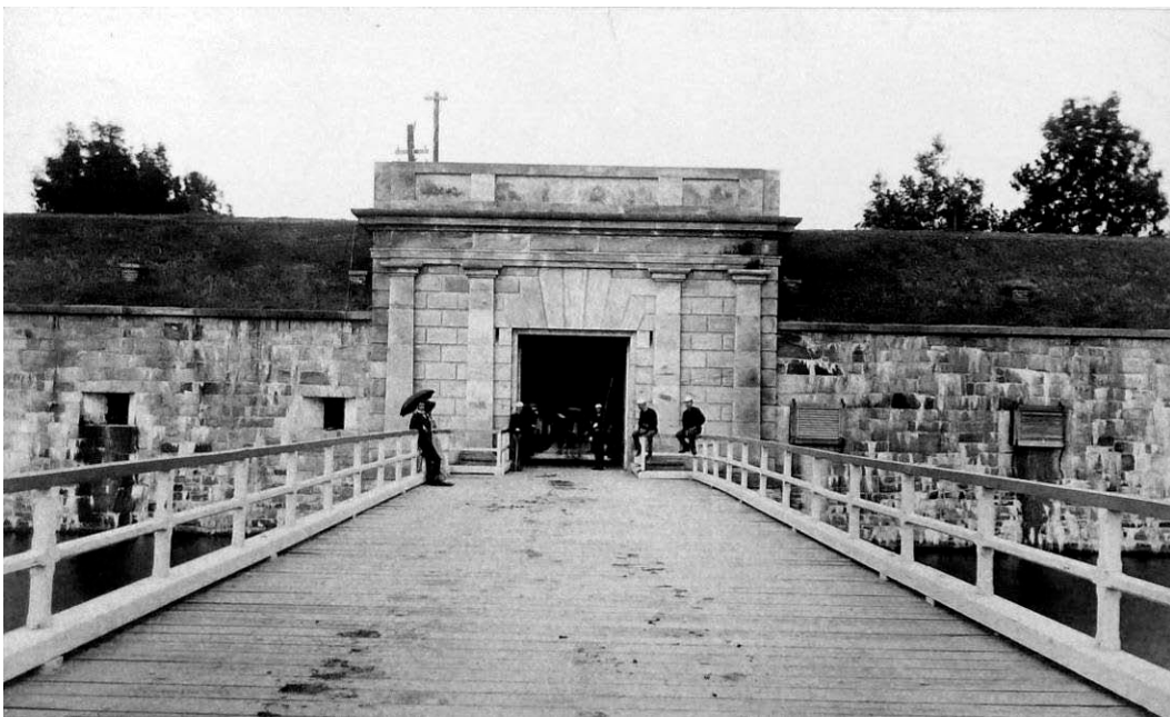
Figure 250: Main gate (NARA 165-FF Box 9B, 20-21).
