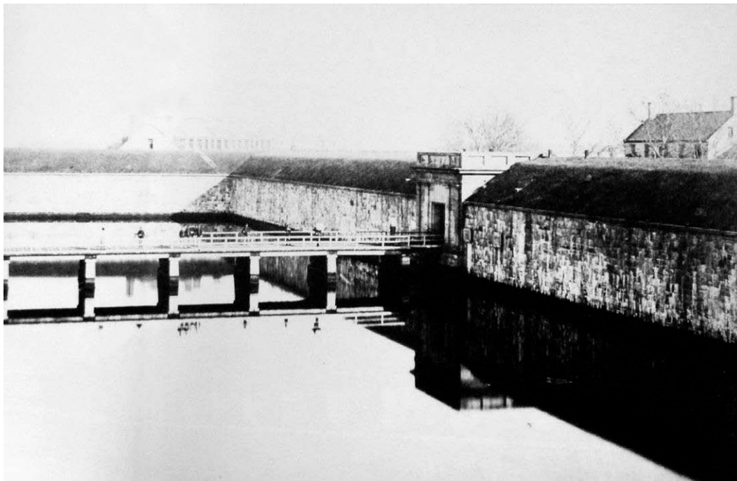
Figure 220: Main Sally Port (NARA 165-FF Box 9B, 20-21).
