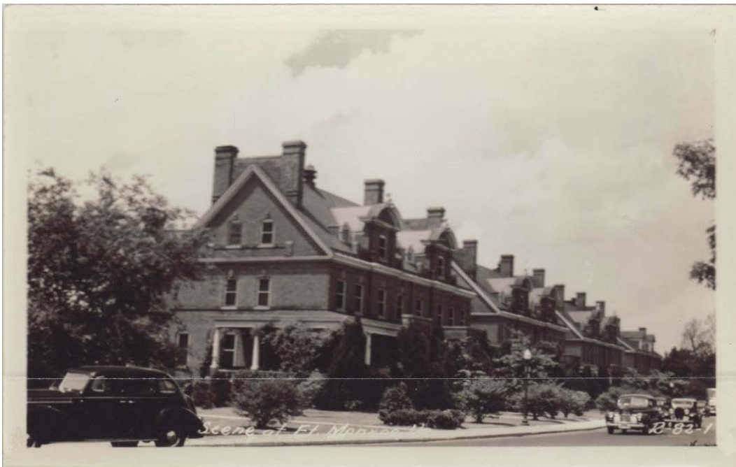
Figure 127: Post Card of Officers' Quarters along Ingalls Road (Casemate Museum).
