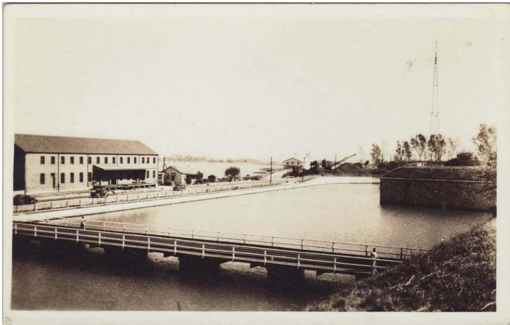
Figure 131: Post Card of North Gate (Casemate Museum).
