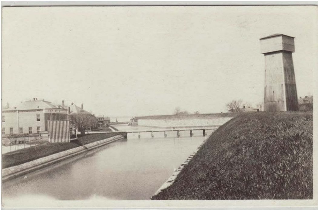
Figure 132: Post Card of Main Gate (Casemate Museum).
