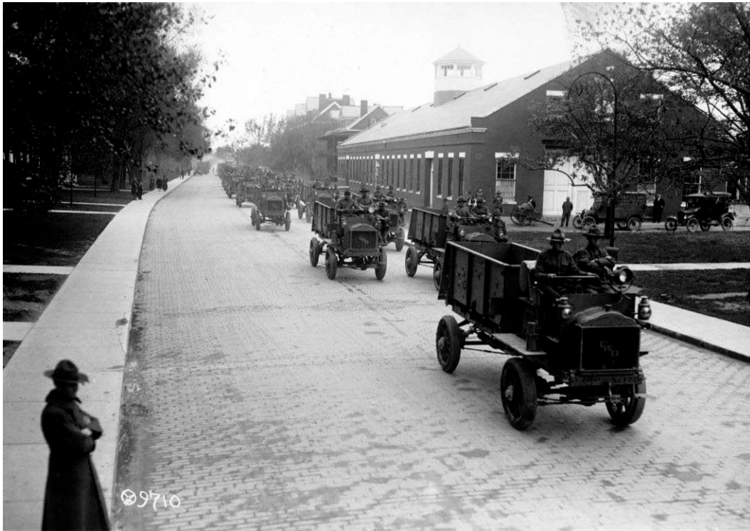
Figure 301: Review along Ingalls Road, 1918 (NARA RG 111-SC Box 68 9710).
