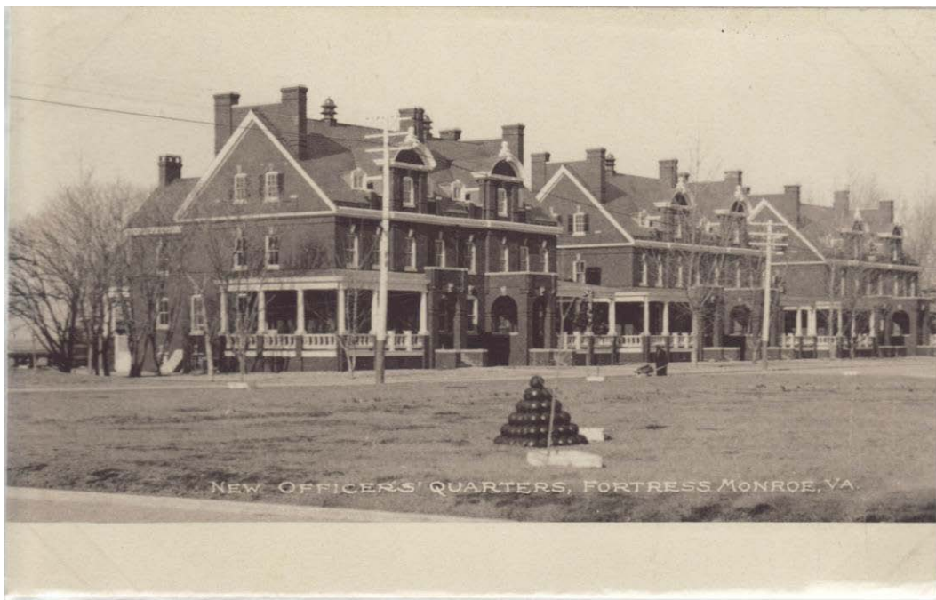
Figure 129: Post Card of Officers' Quarters along Ingalls Road (Casemate Museum).
