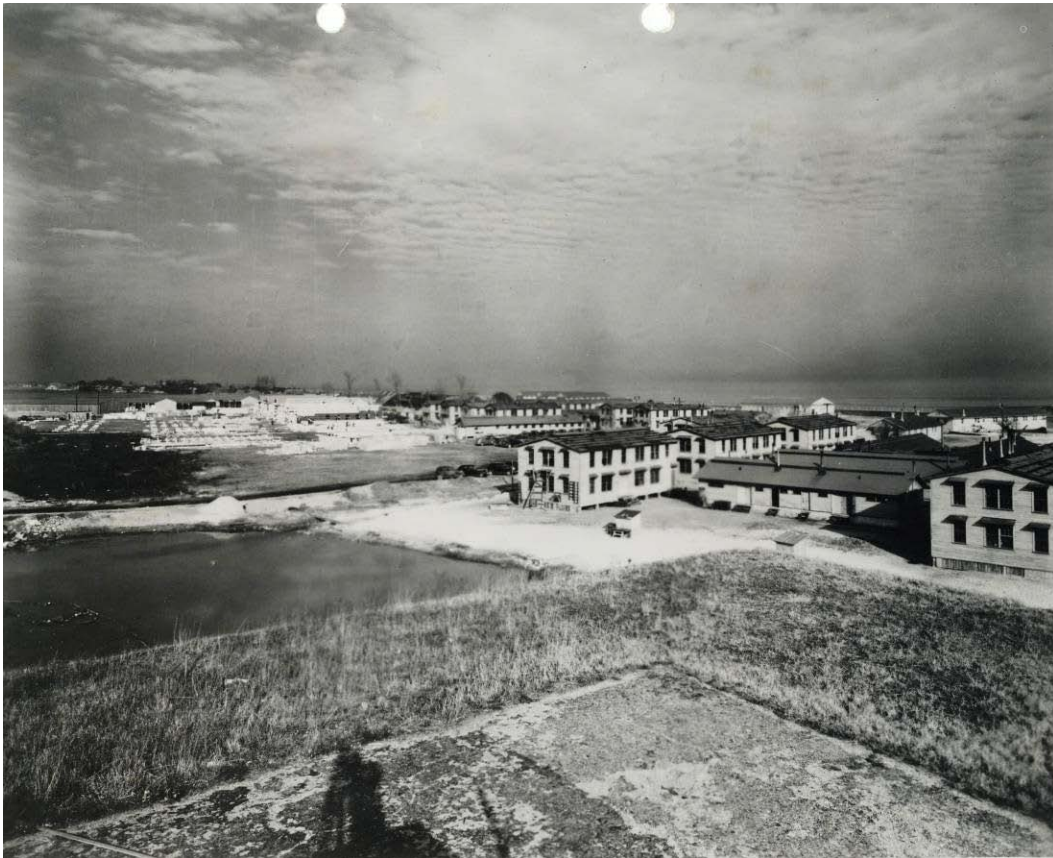
Figure 394: View from northeast bastion, 1941 (Fort Monroe Cultural Resources).
