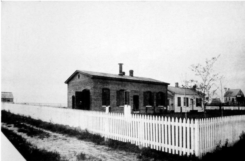
Figure 225: Pumping Station (NARA 165-FF Box 9B, 20-21).
