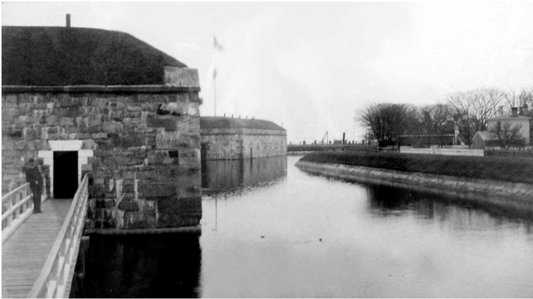
Figure 257: Postern Gate (NARA 165-FF Box 9B, 20-21).
