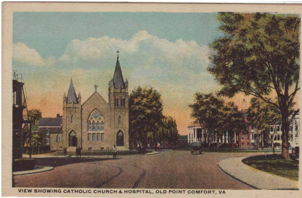
Figure 170: Post card of Catholic Church and Hospital (Casemate Museum).
