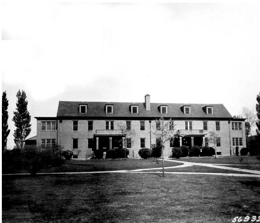
Figure 246: Student Apartments (NARA 165-FF Box 9B, 20-21).
