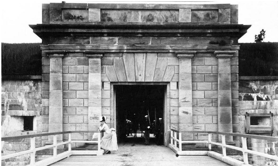
Figure 251: Main Gate (NARA 165-FF Box 9B, 20-21).
