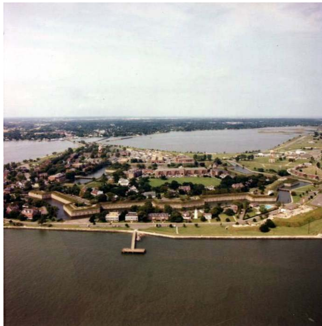
Figure 344: Aerial View 25 May 1982 (NARA).
