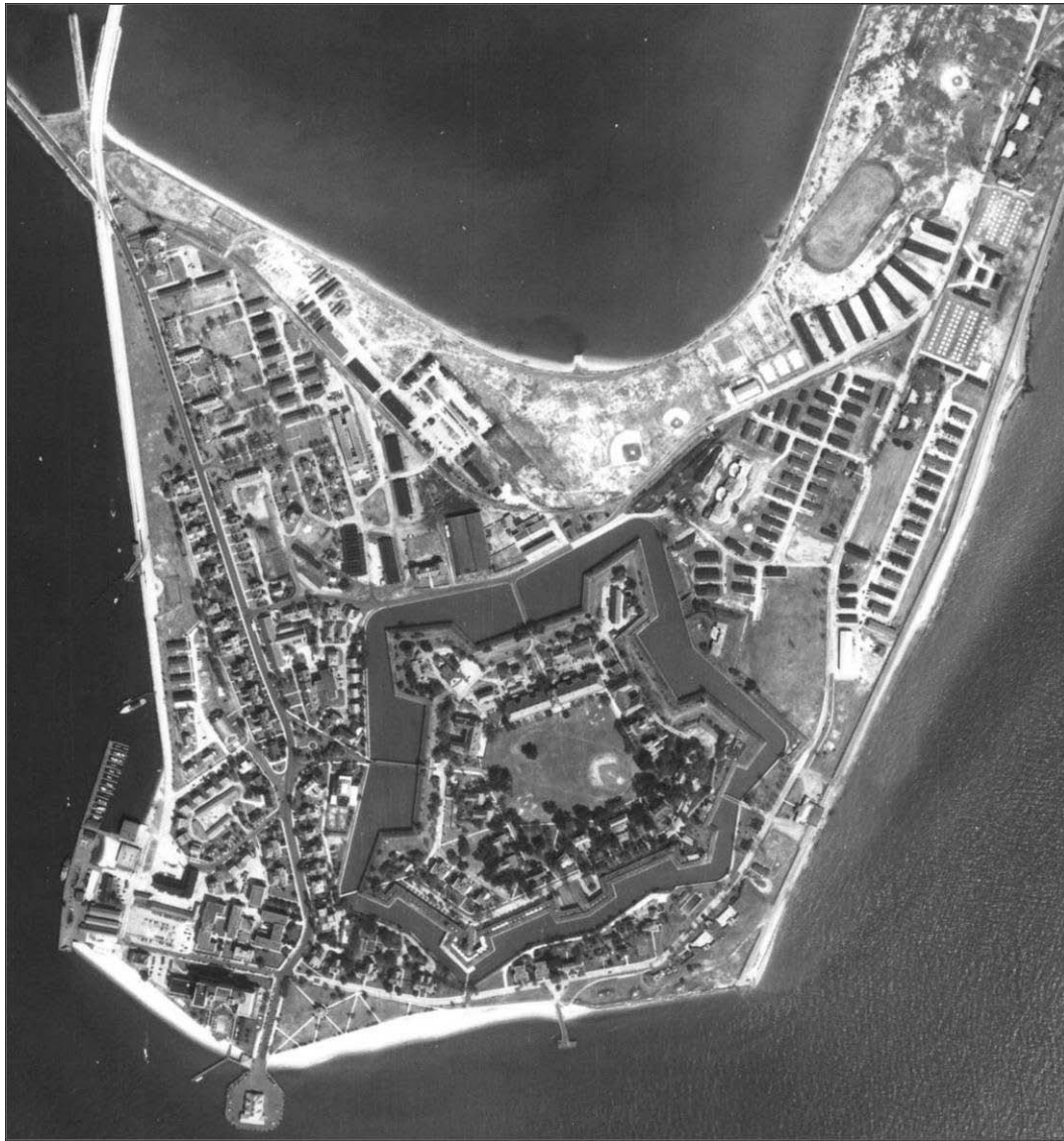
Figure 401: Aerial View of beaches near Baltimore Wharf, 1948 (Fort Monroe Cultural Resources).
