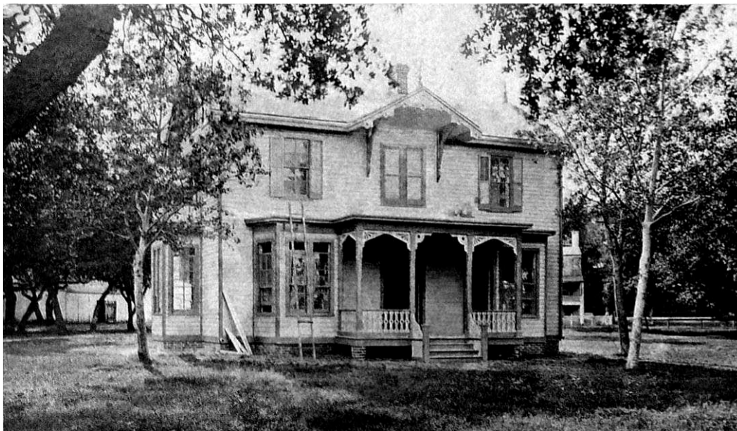
Figure 214: Company Officer's Quarters adjacent to Parade Ground (NARA 165-FF Box 9B, 20-21).
