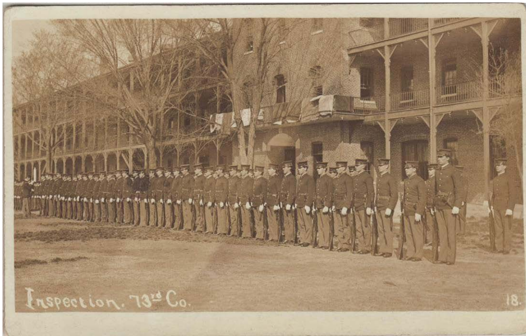
Figure 152: Post card of Building 5 along Parade Ground (Casemate Museum).
