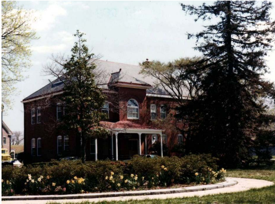
Figure 339: 7-3-Post Headquarters 5 Apr 1978 (NARA CC 107388).
