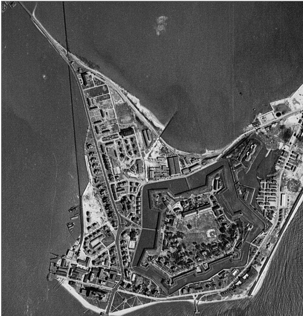
Figure 399: Aerial view before fill along north shore, 1937 (Fort Monroe Cultural Resources).
