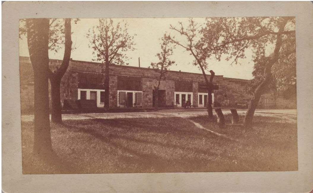
Figure 12: Guard House, 1884 (Casemate Museum, MNRO 6509).
