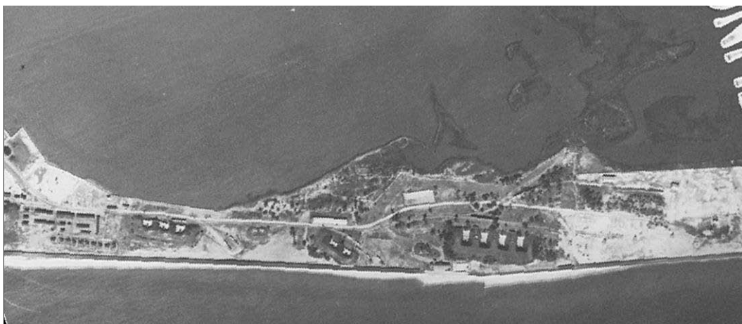
Figure 400: Aerial view, 1937 (Fort Monroe Cultural Resources).
