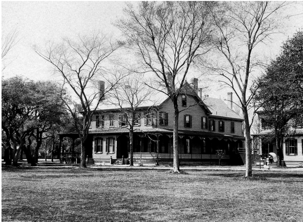
Figure 269: Line Officers' Quarters (NARA 165-FF Box 9B, 20-21).
