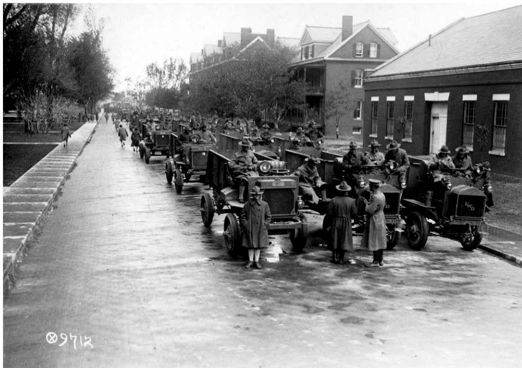
Figure 302: Review along Ingalls Road, 1918 (NARA RG 111-SC Box 68 97012).
