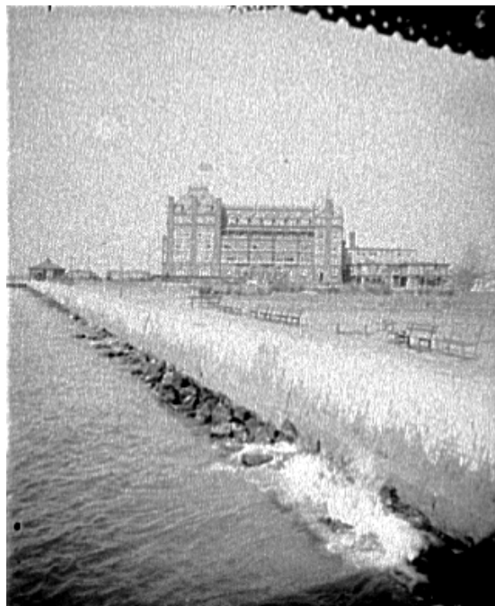
Figure 348: Sea Wall, Old Point Comfort, c. 1900-1915 (LC-D4-15675).
