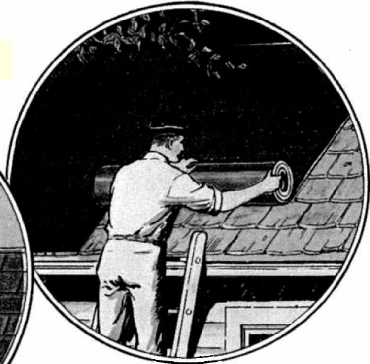
Re-Roofing Over Old Wood Shingles
