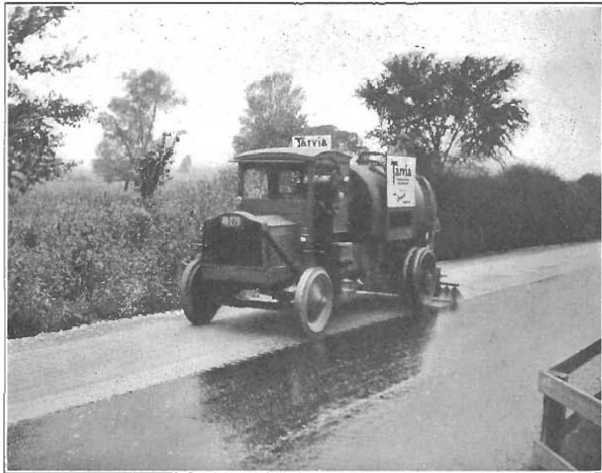
Applying Seal Coat
