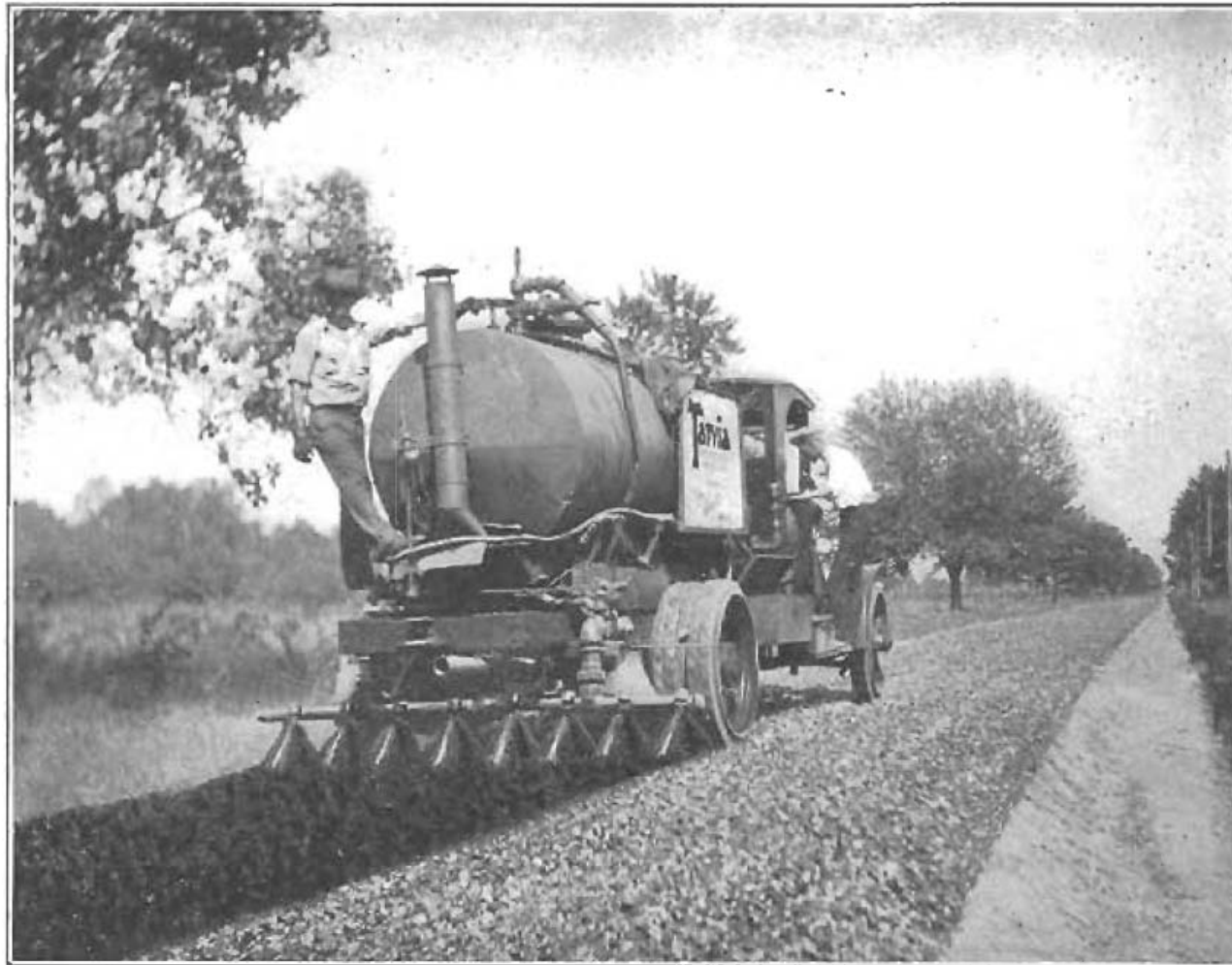
Applying Tarvia Re-Tread
