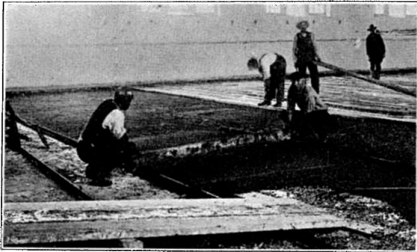
Installing damp-proof course Tar-Rok First Floor, St. Joseph's School Cleveland, Ohio
