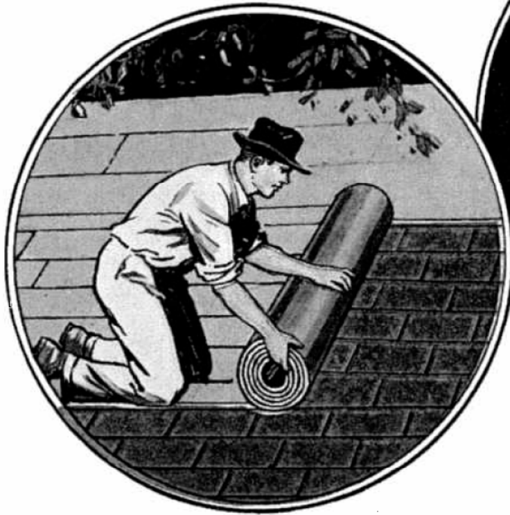
New Roof Decks
