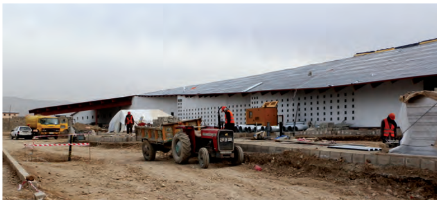
Gardez hospital under construction. (SIGAR photo)
