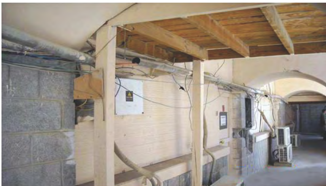
Figure 2. Noncontiguous Raceway in Outdoor Location
