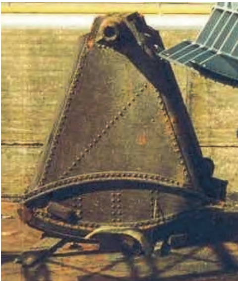
Figure 3. Original reverse tainter valve
