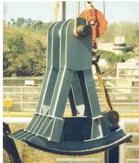
Figure 4. Replacement reverse tainter valve.
