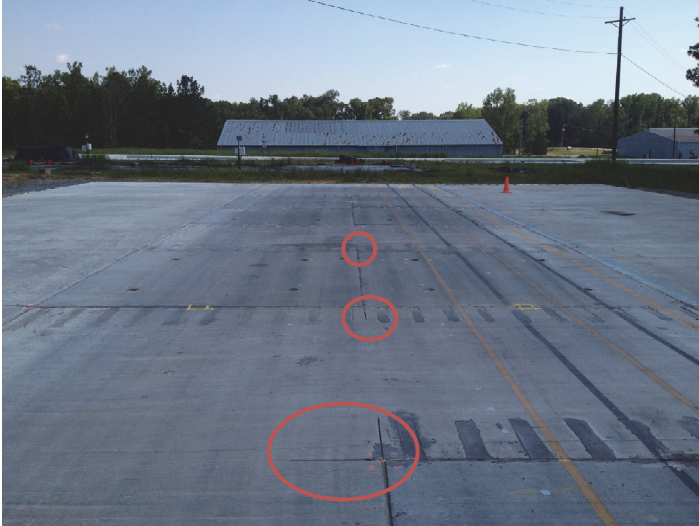
Figure 12. Saw cuts at corners of panels.
