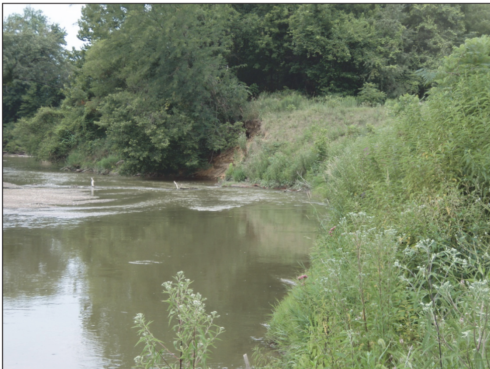
Figure 2.11. Yellow River bank erosion occurring upstream of Knox, IN.
