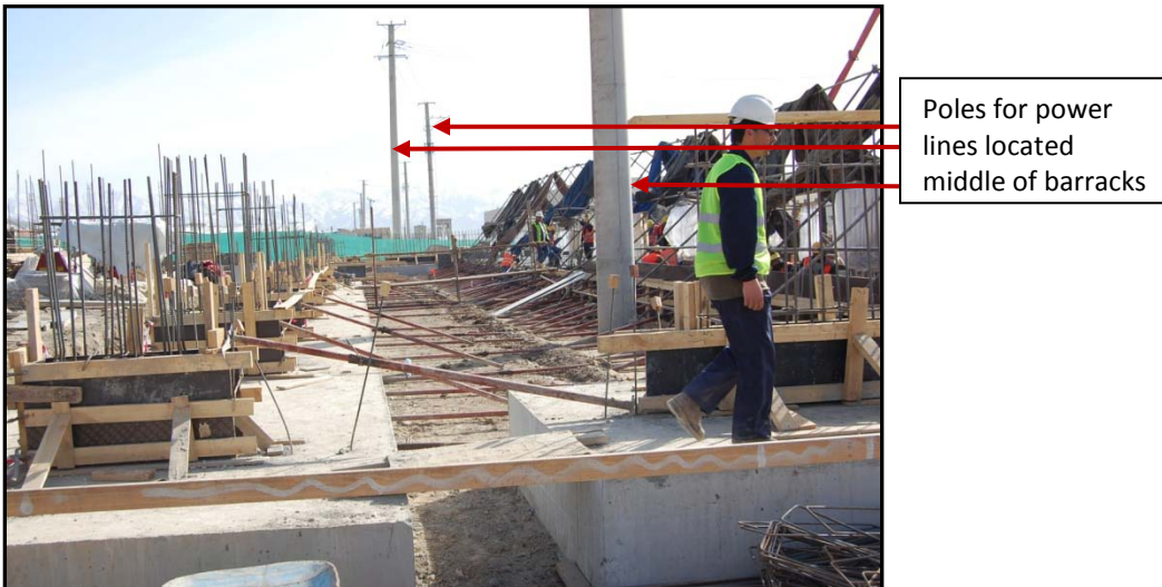
Photo 4: KMTCC Phase III Construction Site
