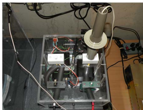
Modified Power Supply Transformer Box
