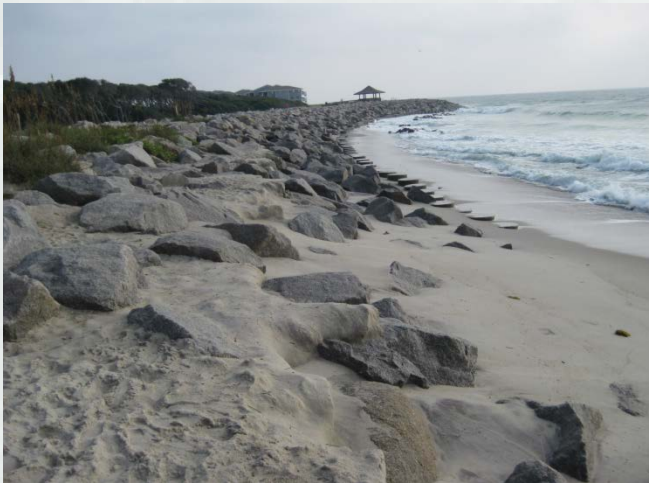
Fort Fisher Revetment
