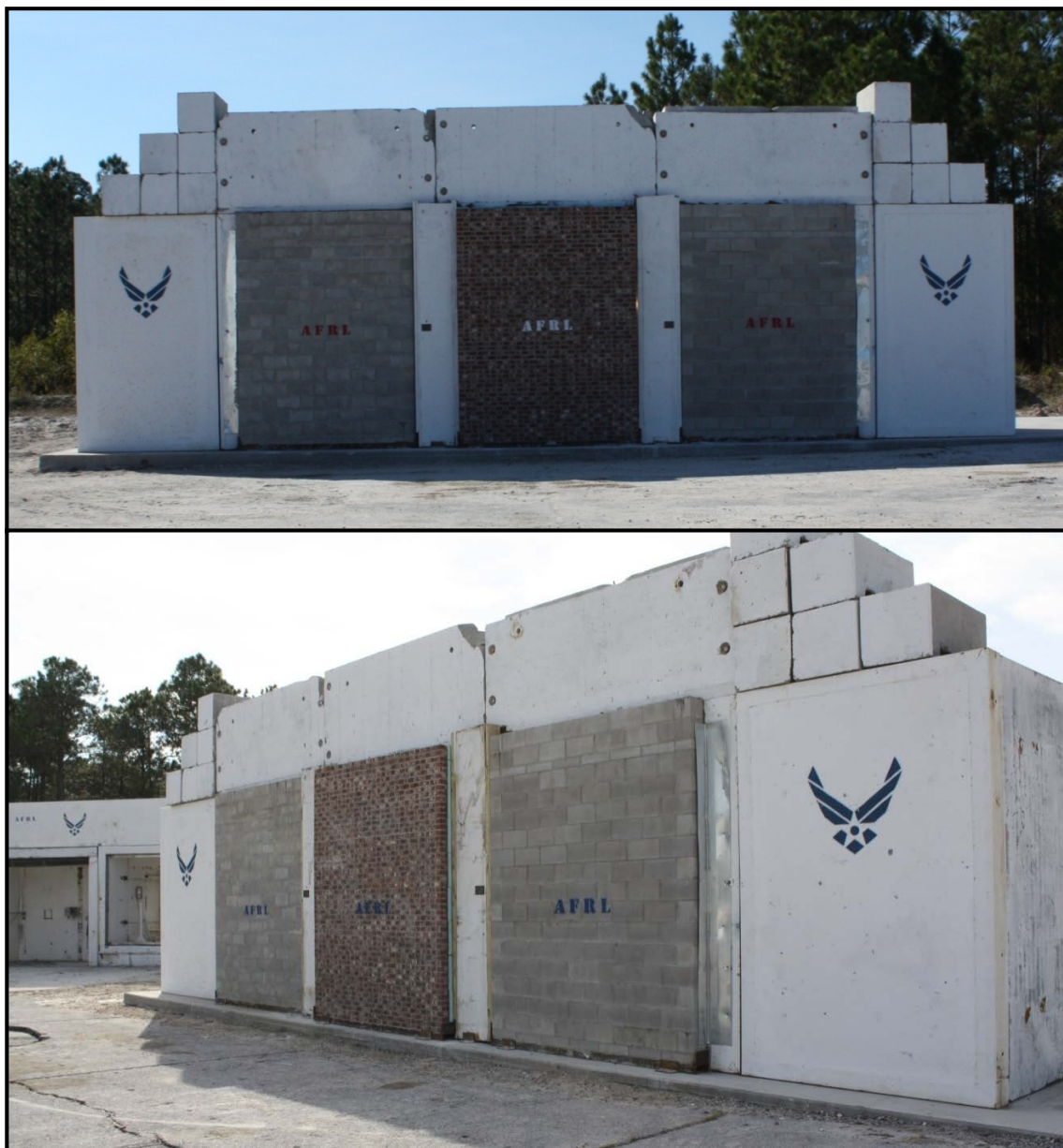
Figure 4. Panels in Reaction Structure Prior to Testing
