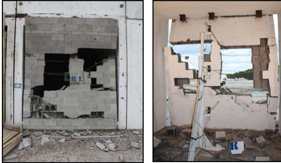
Figure 6. Breached 8-in CMU Wall after Test 2
