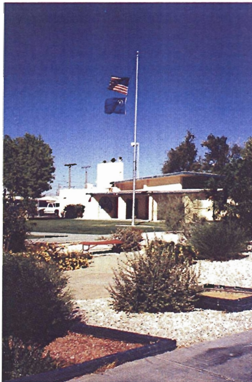
Photograph C-4. Lomie Heard Elementary School. View looking north.
