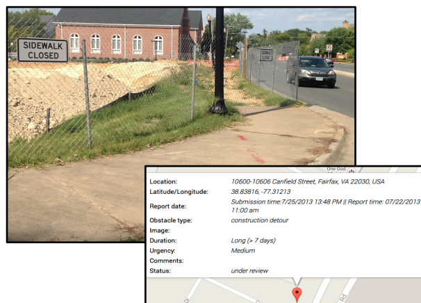
Figure 20. Sidewalk closed and detour into roadway, reported by contributor application, Obstacle Location menu
