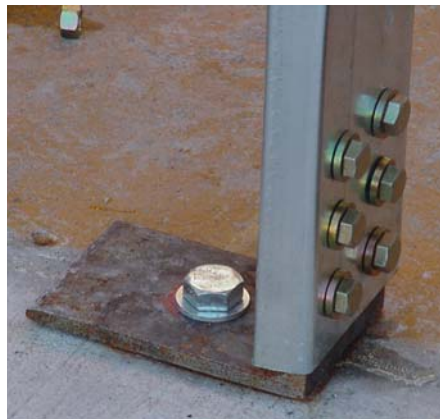
FIG. 3. Stud-to-floor anchorage using a \frac{1}{2} "-thick steel angle
