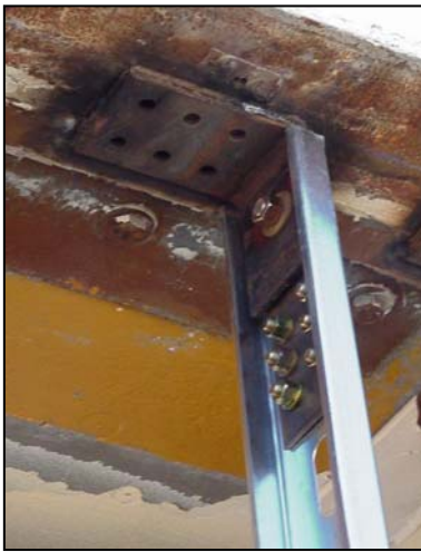
FIG. 8. Connection detail at top of stud showing attachment to embedded steel plate
