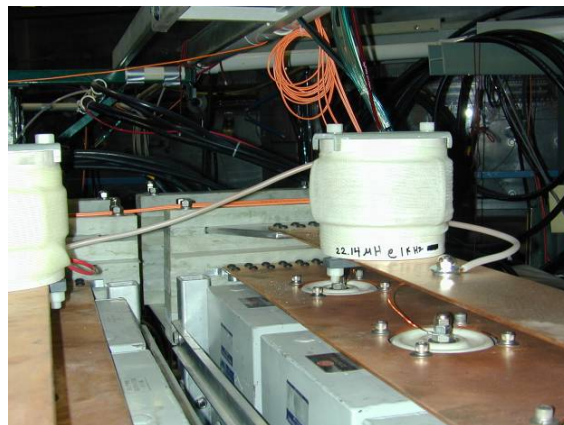
Figure 137. New inductor between Guide/Mirror modules 2 and 3
