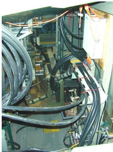
Figure 18. Trigger and charging cables on new cable tray
