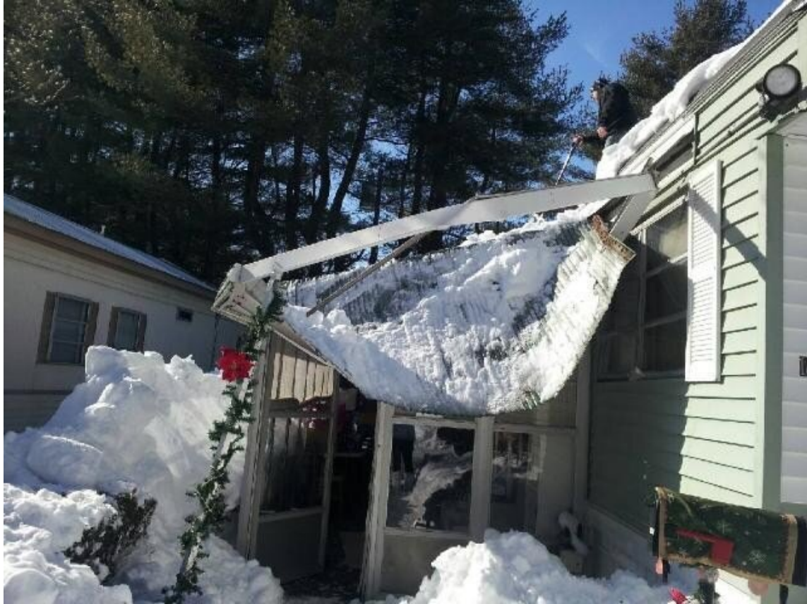
Figure 19. Picture uploaded to Twitter by @SNEWeather, found in the popular retweet, “RT @MassEMA: Why roof clearing is important: MT @SNEWeather partial roof collapse at house in Marlborough Mass http://t.co/8hJb7YlD #MAstorm.” 204,205
