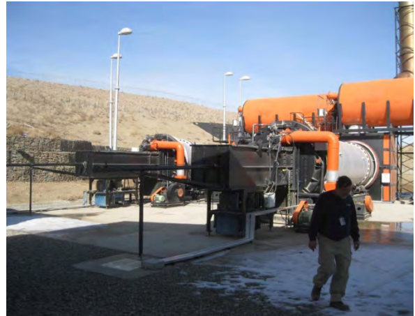
Photo 2 - Loading Area for Incinerators
