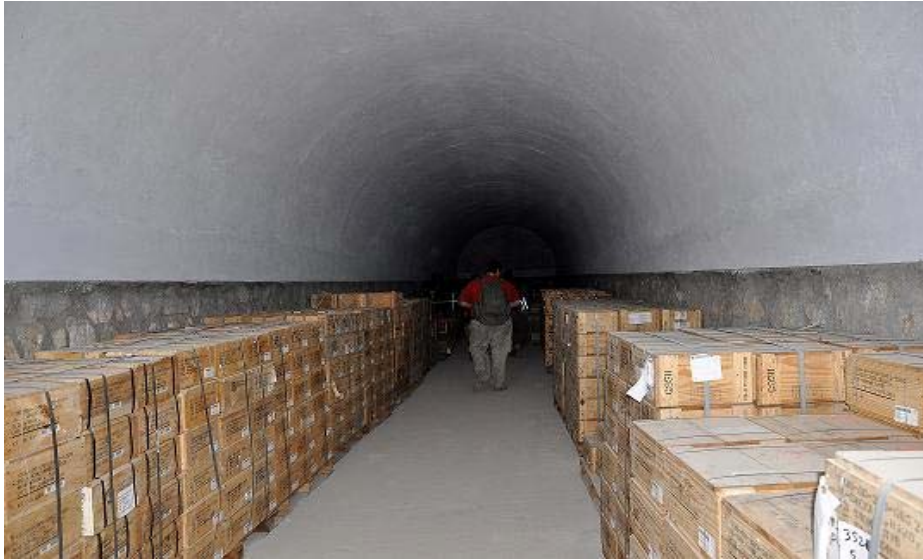
Figure 7 – A member of the assessment team inspects ammunition at 22 Bunkers
