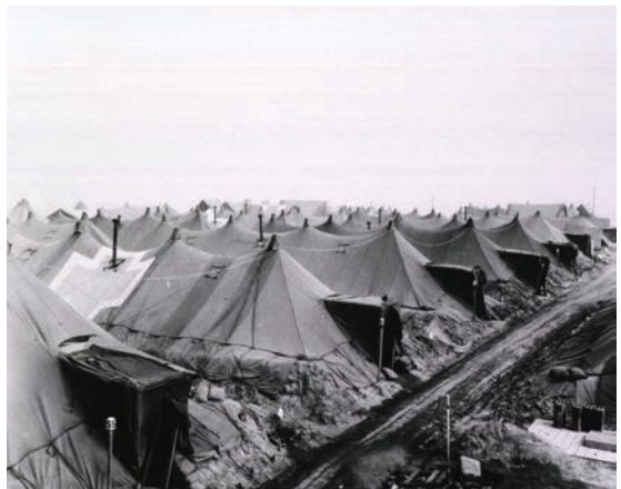
May 8, 1944, Anzio, Italy: The sides of the ward tents of the 94th Evacuation Hospital were reinforced with earthworks.
