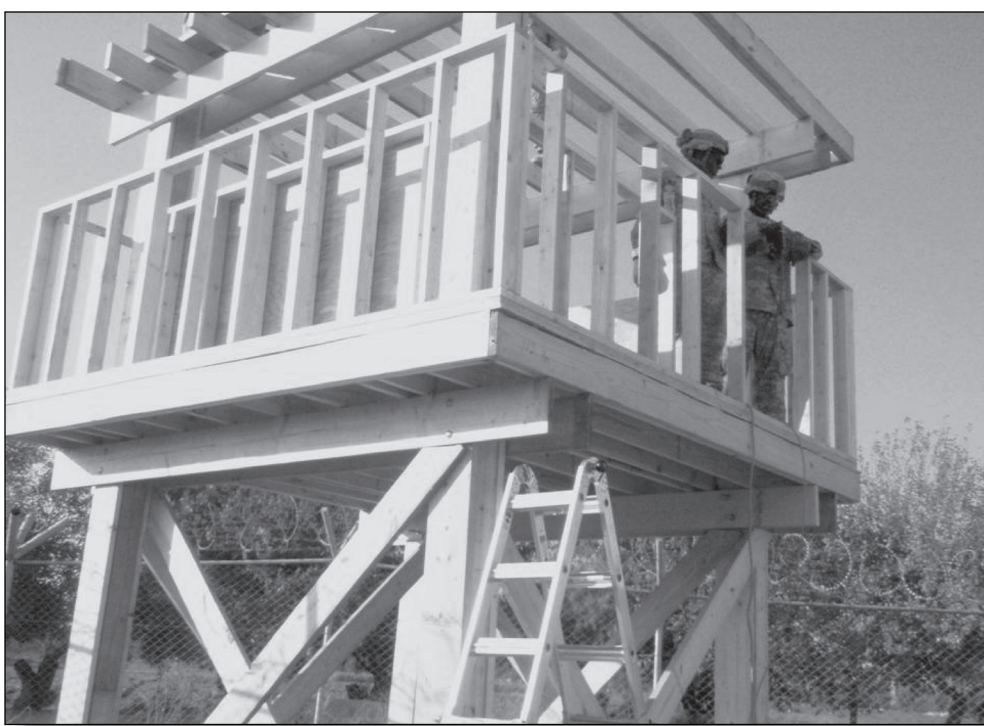
Standard Guard Tower Construction
