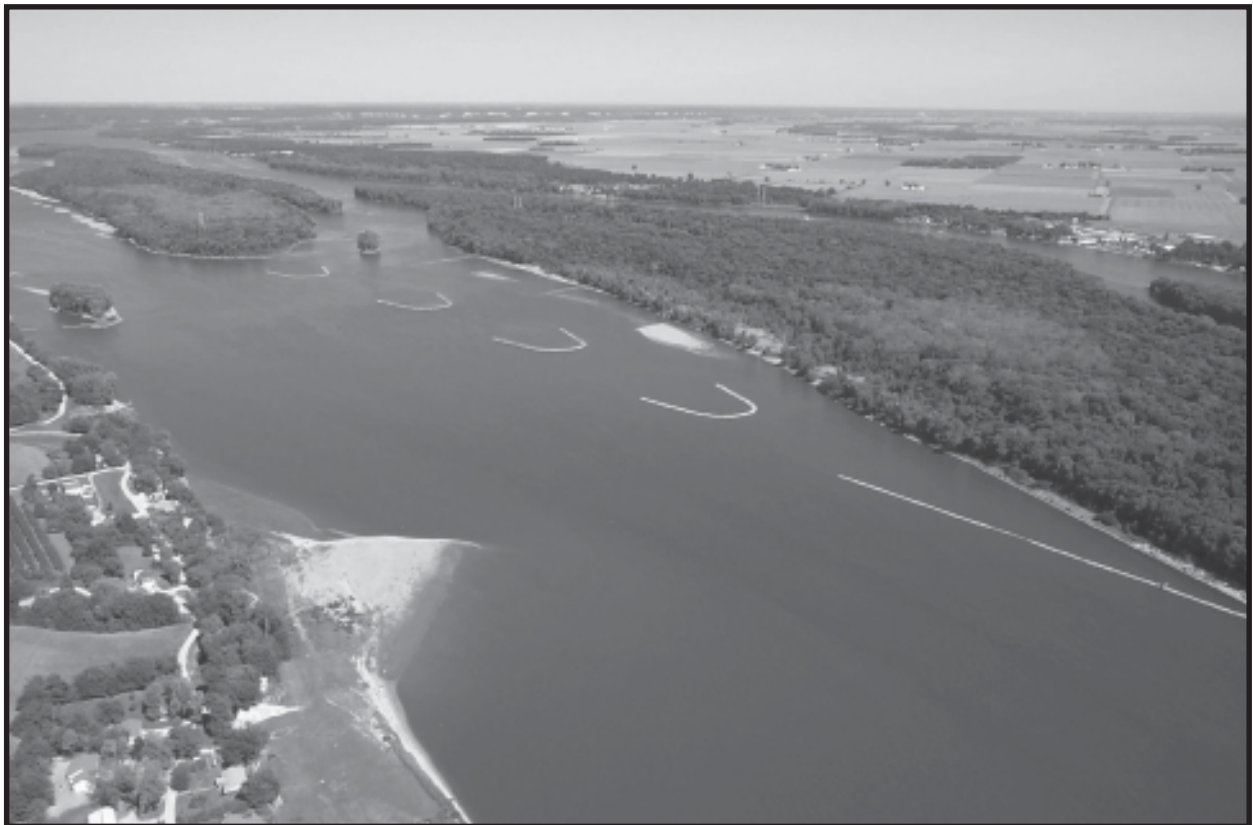
Innovative river training structures remedied a chronic dredging problem and created unique aquatic habitat.
