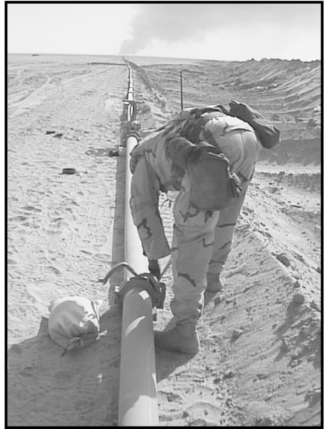
A soldier from the 62d Engineer Battalion couples a section of the pipeline while an oil fire burns in the background.
