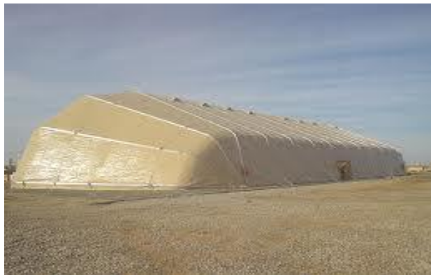
Figure 2. Large Area Maintenance Shelters
