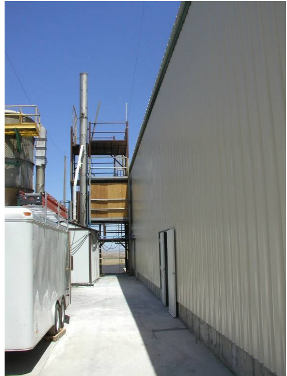
Figure 7. West outside wall of enclosure.
