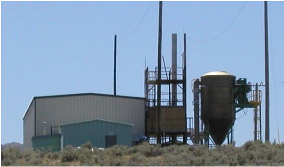
Figure 6. Outside view of North side of enclosure.
