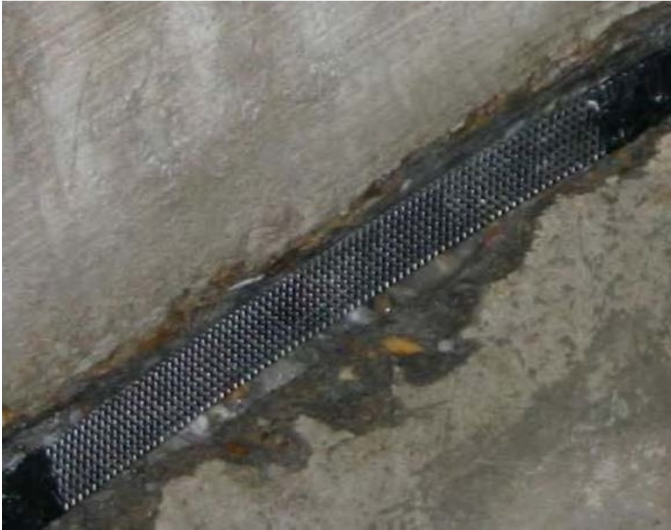
Figure 4. Photograph of anode ribbon installed in basement.
