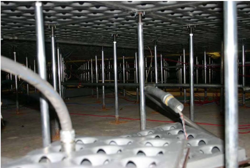
Figure 1. Space below raised panel floor in Hays Hall basement.
