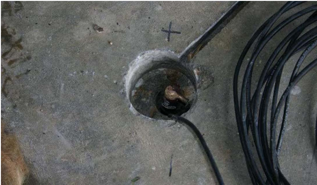
Figure 6. Cathode connection with exothermic weld.
