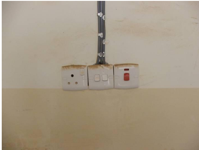
Site Photo 8. Switches
