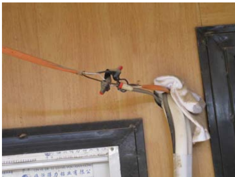
Figure 13. Spin Boldak: A sock used as an electrical insulator and an exposed splice is a fire hazard.
