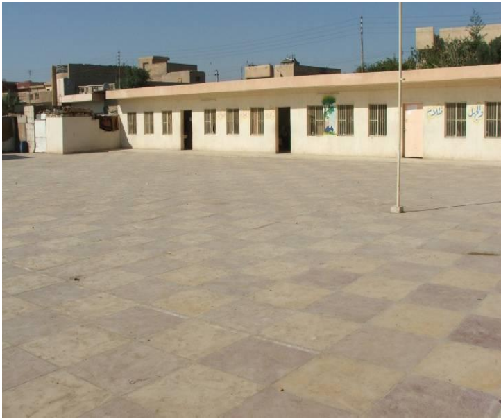
Site Photos 5. New walkway tiles
