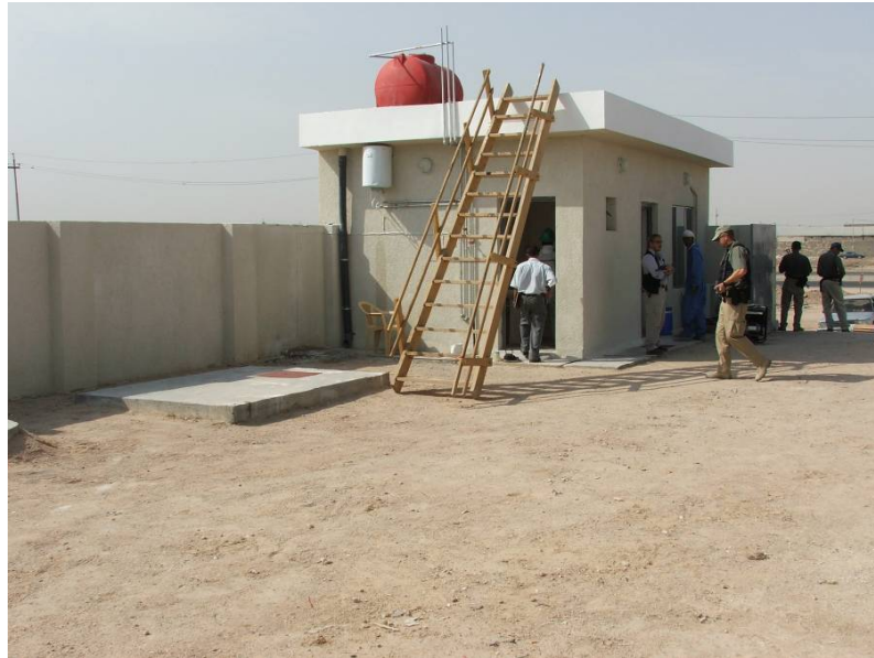
Site Photo 2: Exterior fence, guard house, and gate
