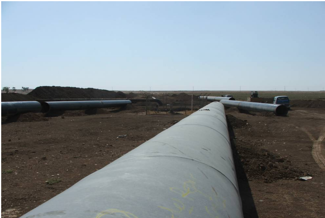
Site Photo 1: Pipes Purchased By Prior Contractor
