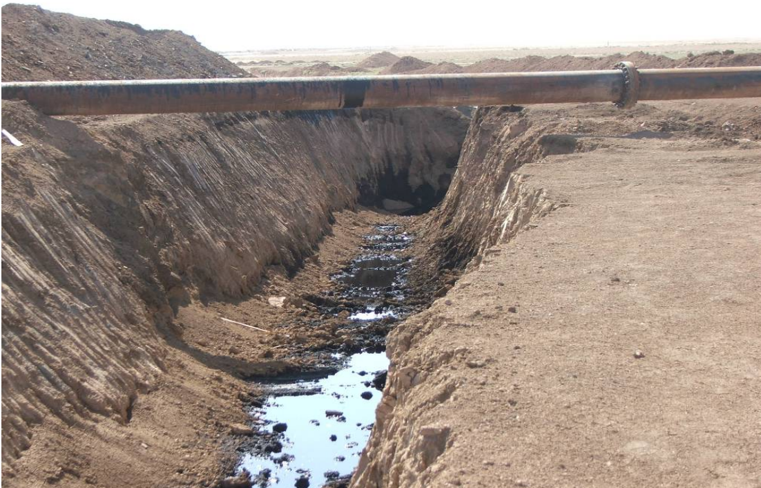
Site Photo 5: Common Example of Pipeline Excavation with Oil Seepage
